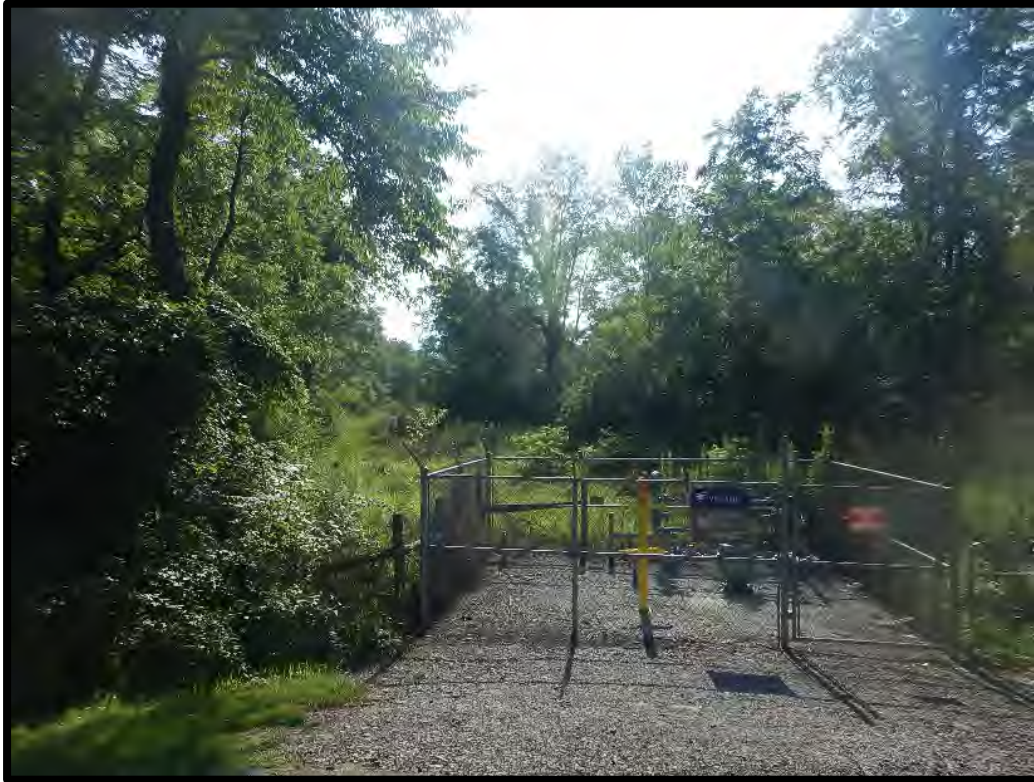
Figure 7. View of the existing gas pipeline in the project area.
