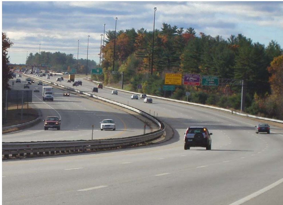
Figure 7 – Southbound Horizontal Curve In Advance Of The Hooksett Tolls
