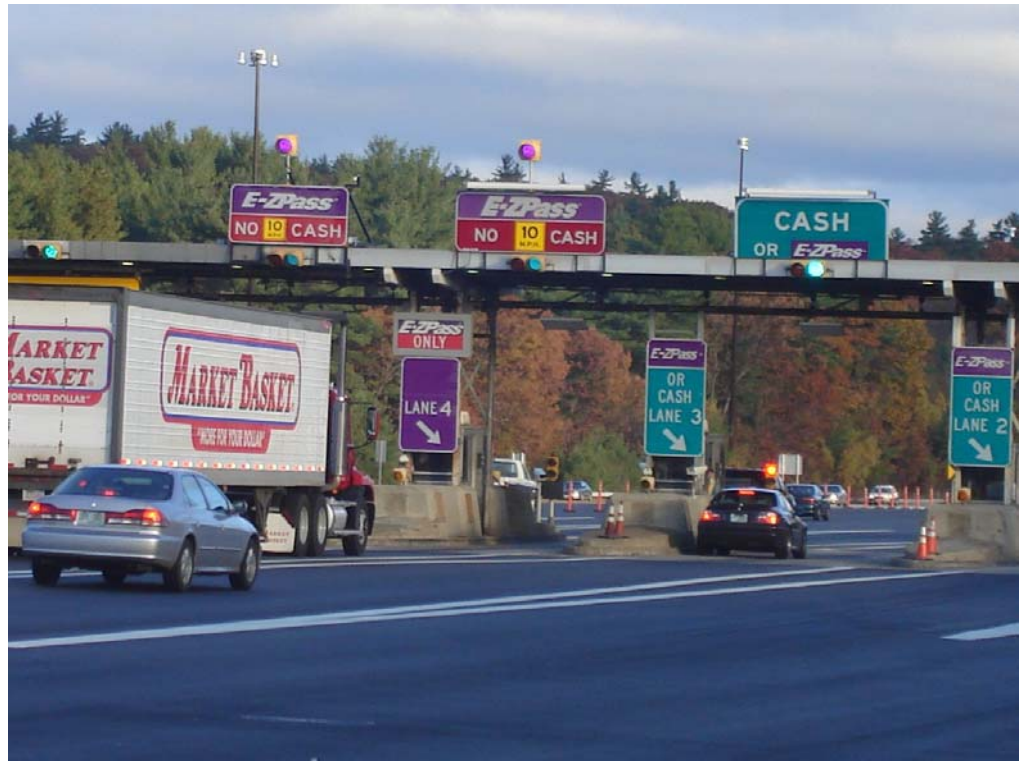
Figure 8 - Installation and Application of Purple Wayfinding Lights
