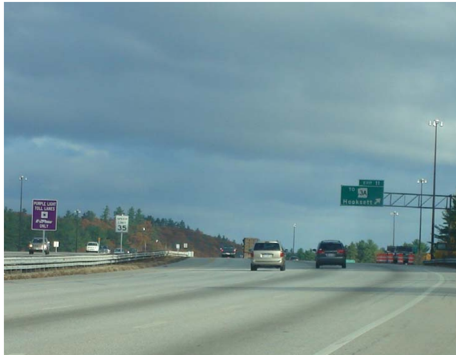
Figure 5 - Northbound Crest Vertical Curve In Advance Of The Hooksett Tolls
