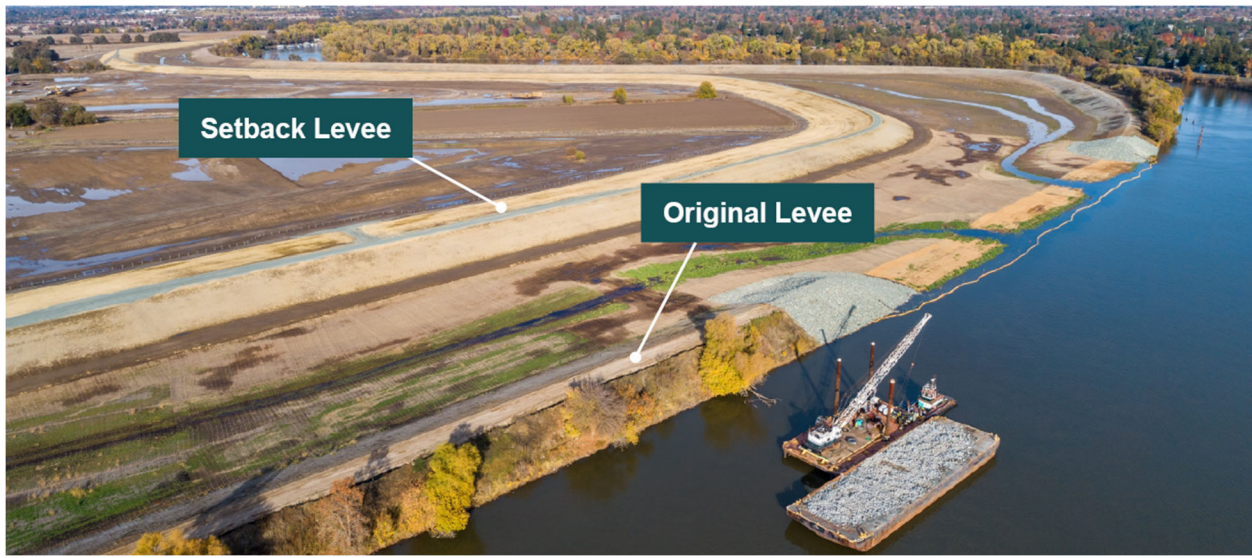
Figure 2-7: Typical Setback Levee
