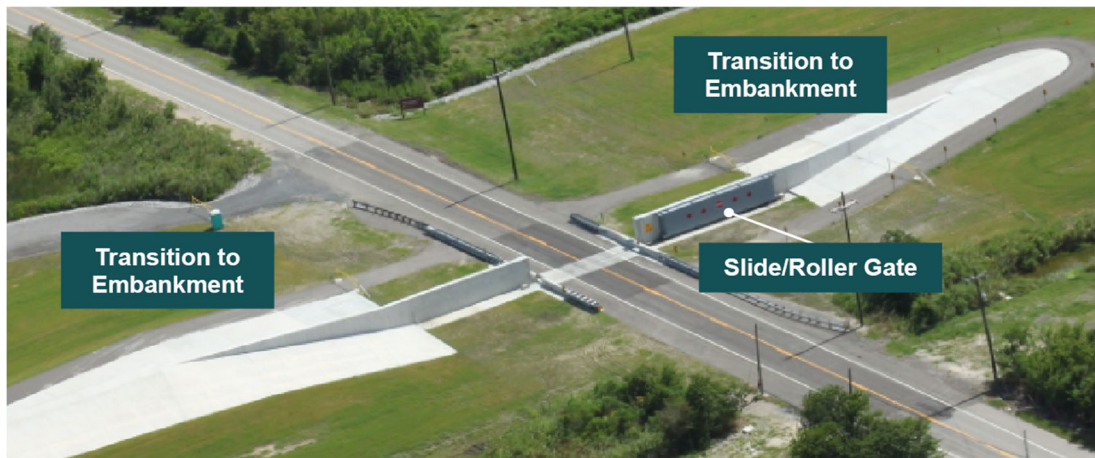
Figure 2-21: Roller/Slide Gate Details
