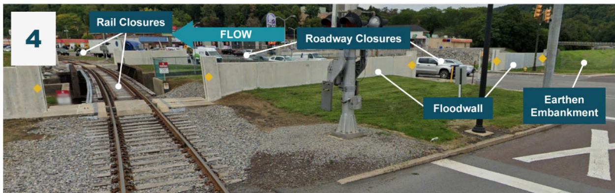
Figure 2-54: Example of Railway and Roadway Closures
