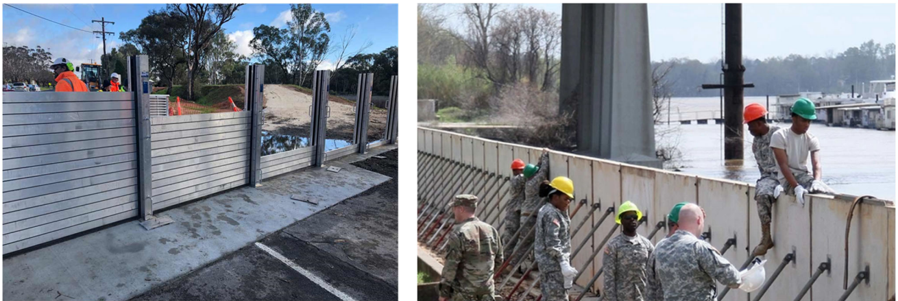
Figure 2-19: Typical Demountable Walls
