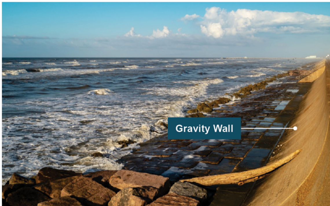
Figure 2-18: Example of Mass Gravity Wall
