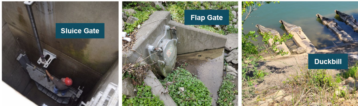
Figure 2-43: Typical Gates for Interior Drainage Systems
