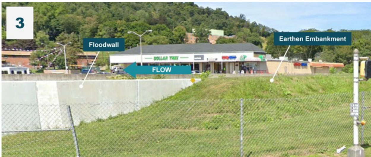
Figure 2-53: Example of Embankment Tie-In to Floodwall
