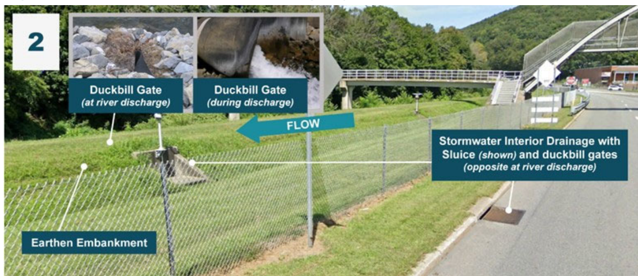
Figure 2-52: Example of Interior Drainage Systems
