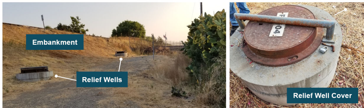
Figure 2-36: Example of Relief Well
