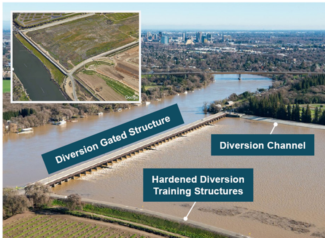
Figure 2-38: Typical Floodway Channel
