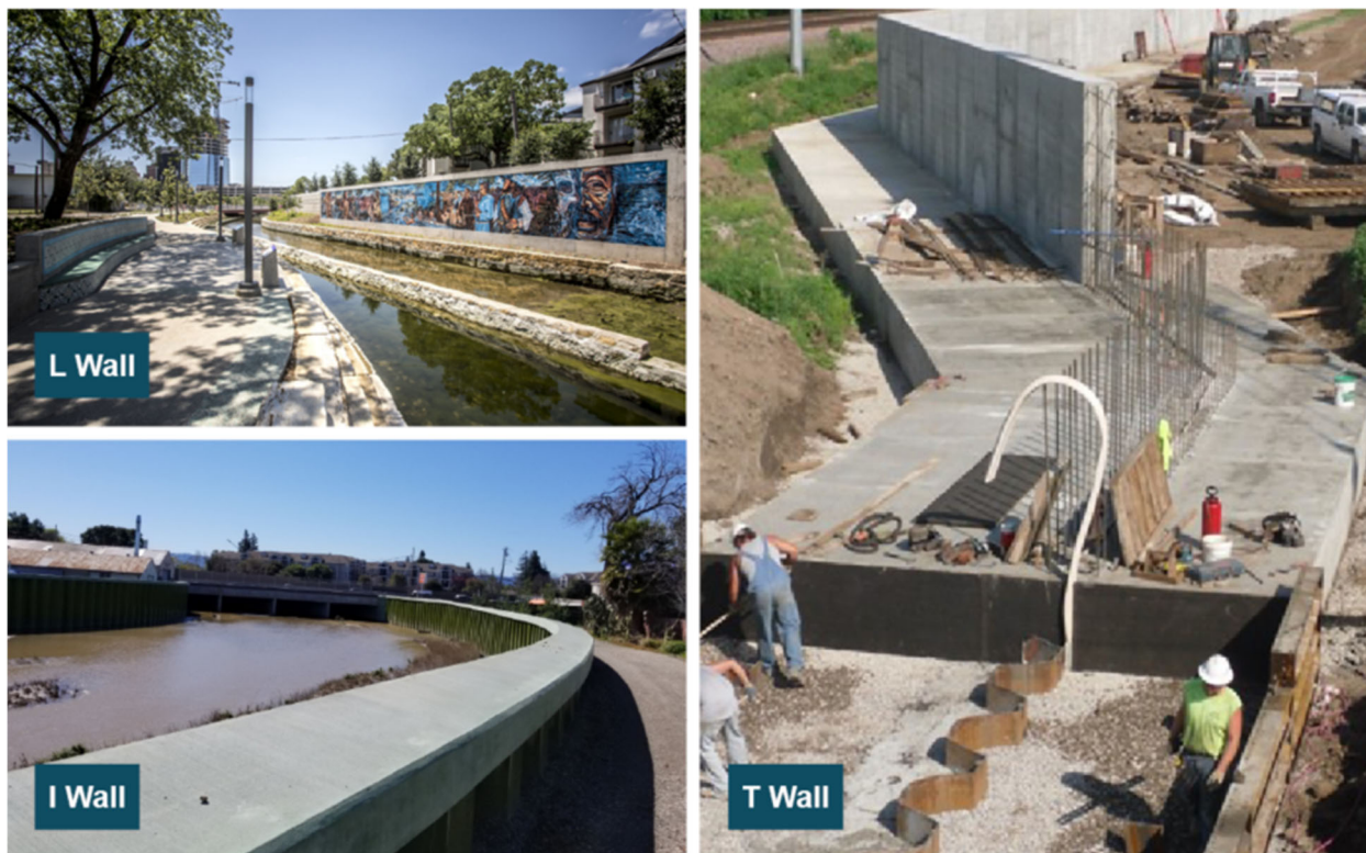
Figure 2-13: Examples of Floodwalls
