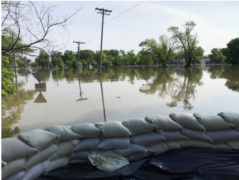
Figure 2-29: Typical Sandbag Closure
