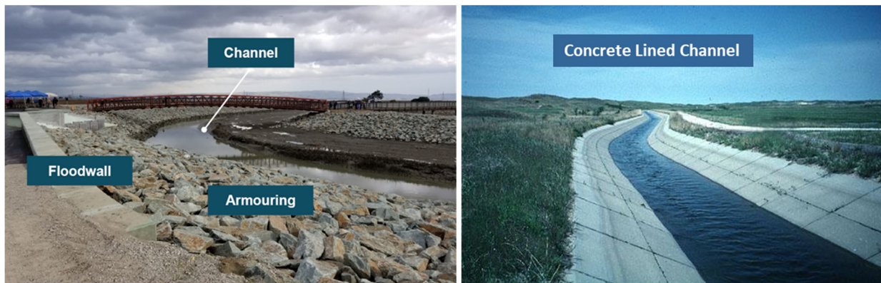
Figure 2-39: Examples of Channel Erosion Control
