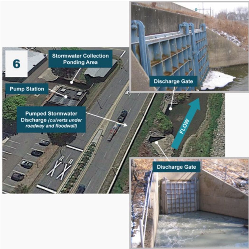
Figure 2-56: Example of Interior Drainage System
