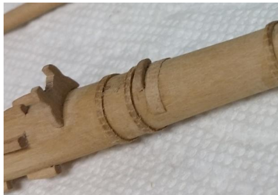
Figure 26 - Spritsail Yard Sling Saddle (and Lead Sheet) Installed to the right (forward) of the Woolding Hoops
