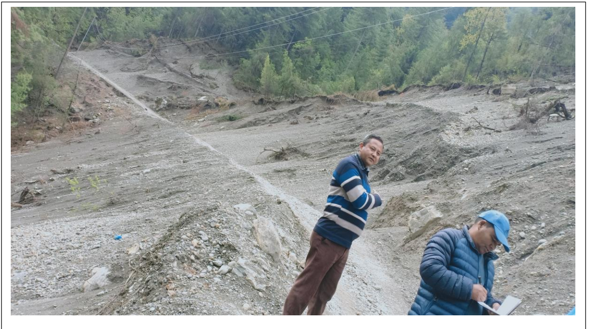
Landslide Hazard: Chame Rural Municipality, Manang
