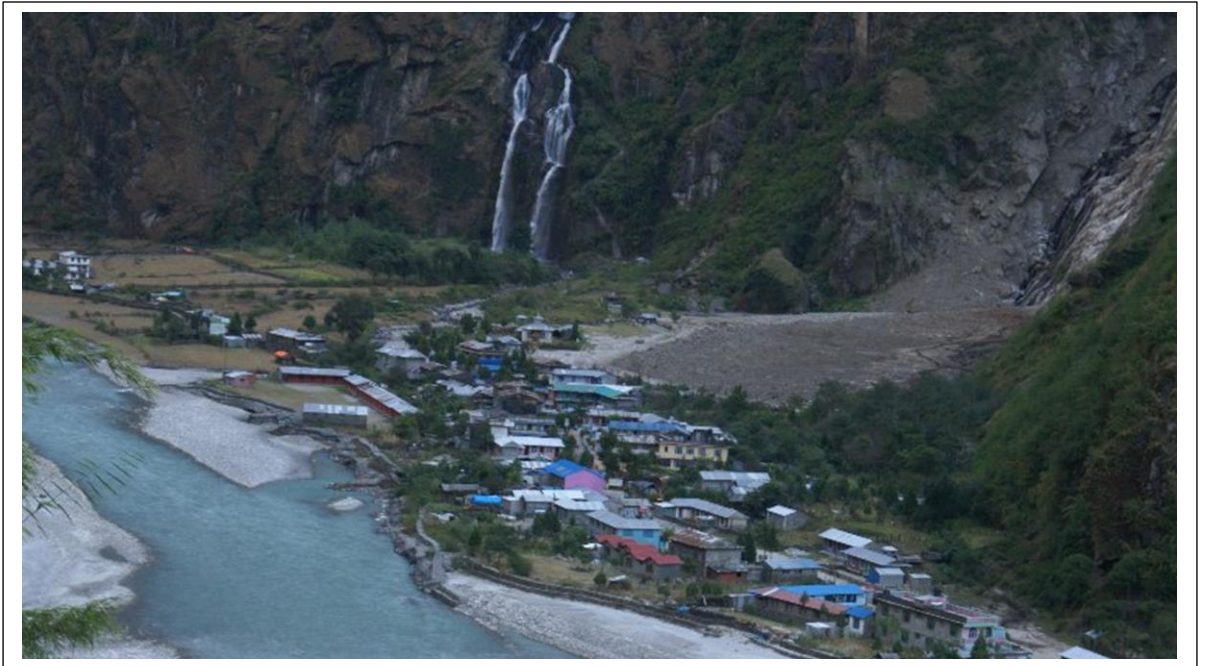
Tal Gaun, Manang: Both, landslide and flood risk hazard
