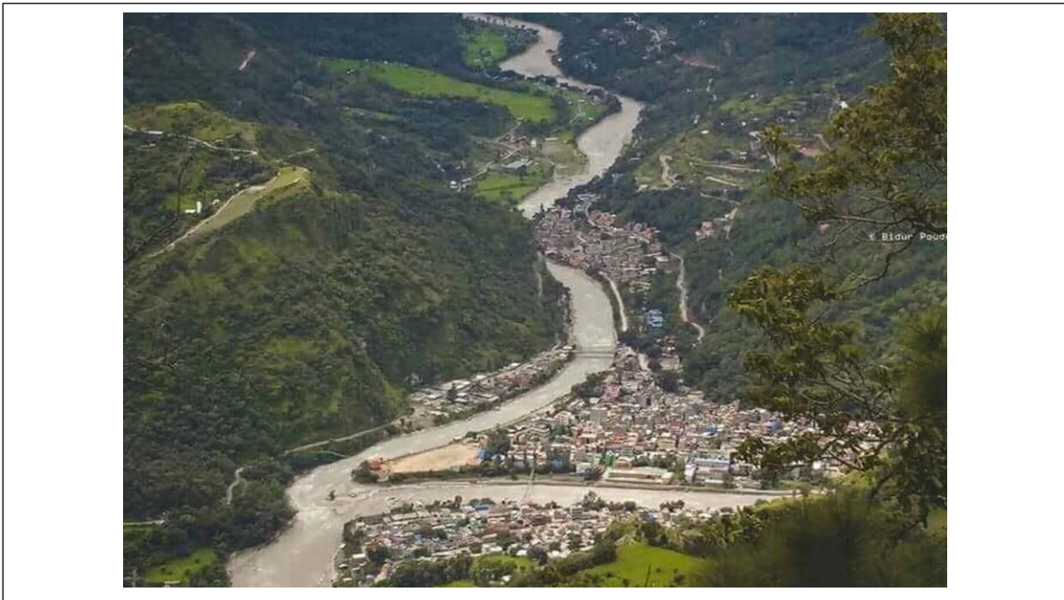
Beni Bazar, Myagdi district: high flood risk area by Kaligandaki River
