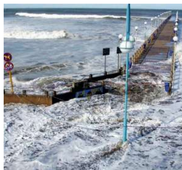
Damage from the March 2007 storm in KwaZulu Natal by high sea-levels and large waves; Top: Beach facilities on the lower South Coast; Middle: Flooding of George Hulett Place, Salt Rock; Bottom: Inundation of North Beach Pier, Durban
