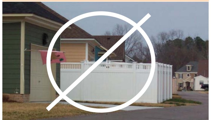
FENCE IS TOO HIGH AND IS INSTALLED OUT OF LEVEL
