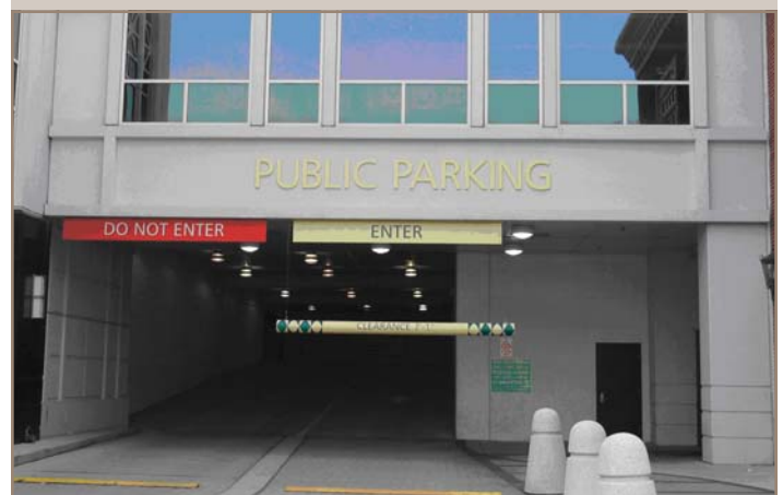
BUILDING IDENTIFICATION SIGNS AT VEHICULAR ENTRY LOCATIONS SHALL BE A MAXIMUM OF 60 SQUARE FEET.
