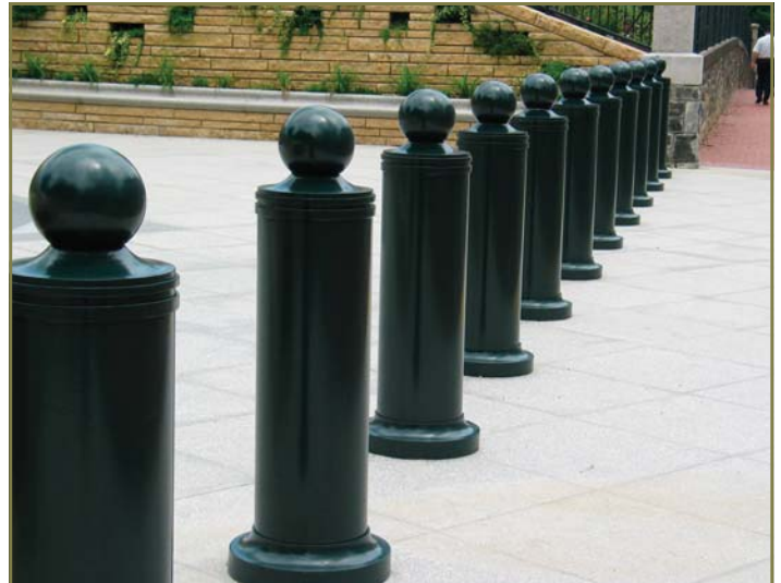
AN EXAMPLE OF STYLIZED METAL BOLLARDS USED TO PROTECT A PRINCIPAL ENTRANCE ALONG A BOULEVARD. METAL BOLLARDS SHOULD BE TREATED TO RESIST THE DETERIORATING EFFECTS OF THE ELEMENTS.
