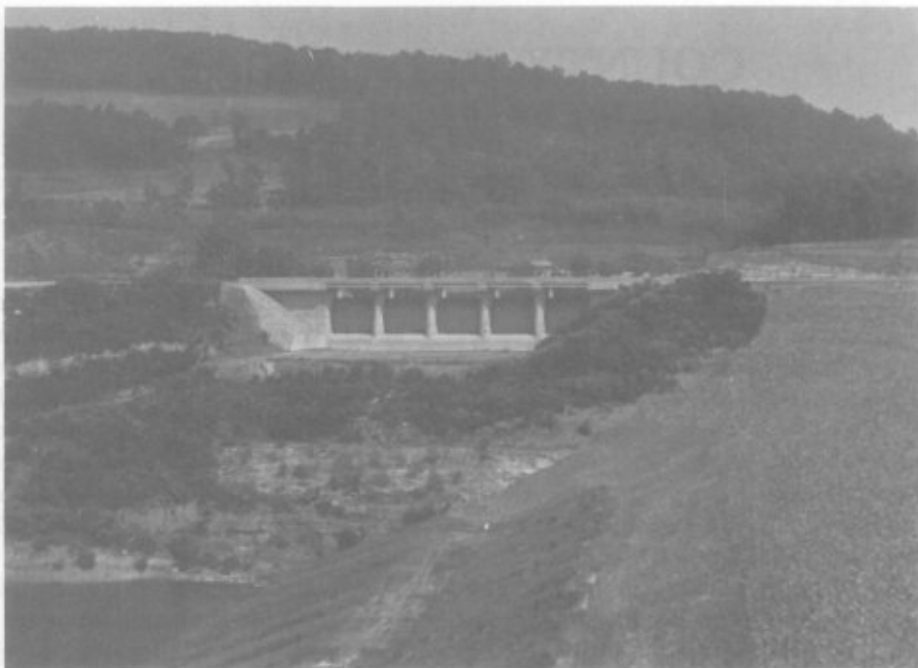
FIGURE 1. The Bloomington Dam
