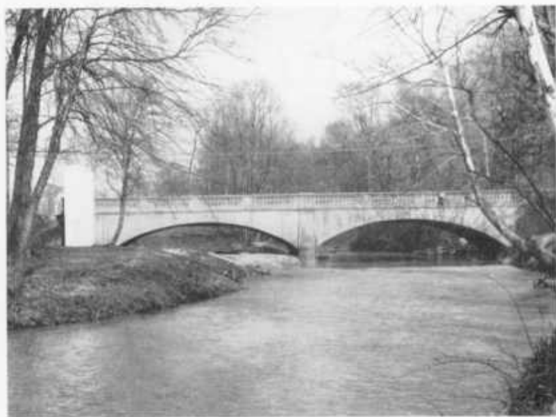
PLATE 1, FIG. 2. Gage House at Stream Flow Measurement Station on Northeast Branch Anacostia River at Riverdale (facing upstream).
