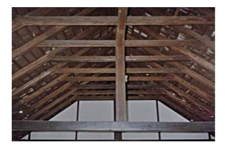
FIGURE 7 Intermediate roof beam and cross-ties at Fort Alice, 1984. (Photograph reproduced with the permission of the Sarawak Museum)
