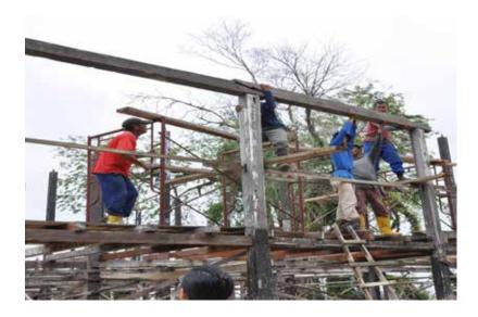
FIGURE 9 Reassembling a hooked scarf connection during Fort Alice's conservation, 2014. (Photograph by the author).
