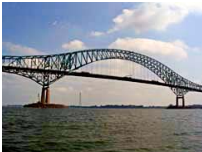
Pont Laviolette (225m horizontal center span with a vertical clearance of 50m)
