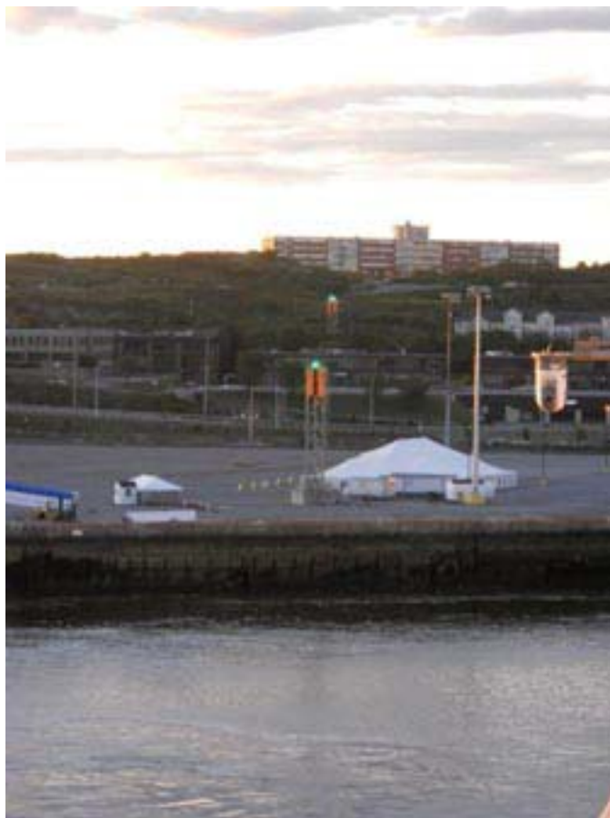
Long Wharf and Long Wharf Range Lights
