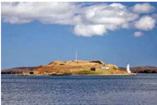
Georges Island—Communication Tower (center)
