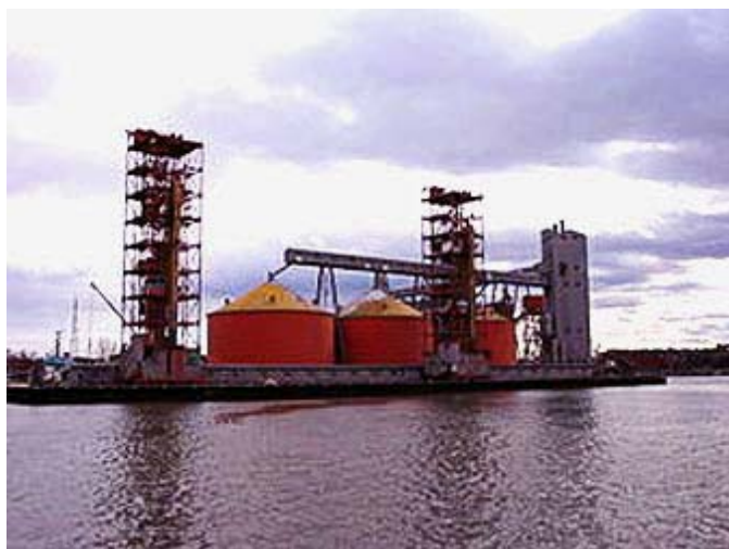
Sorel Wharf—Berths 14 and 15
