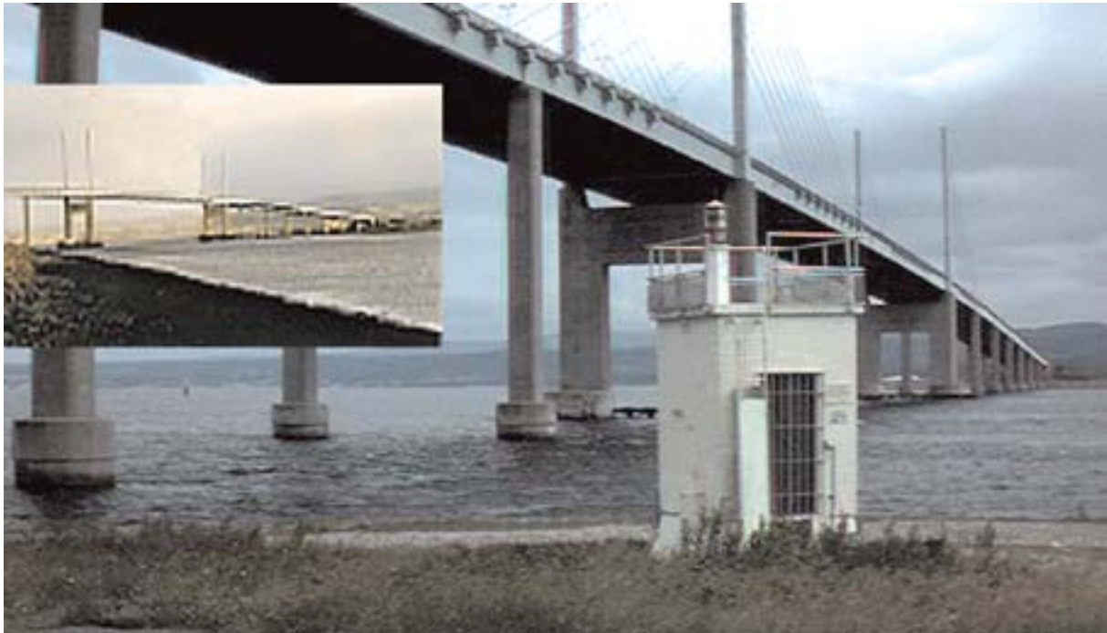
The Kessock Road Bridge
