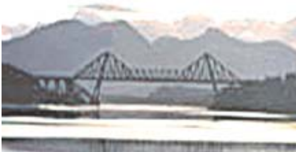
The Connel Bridge
