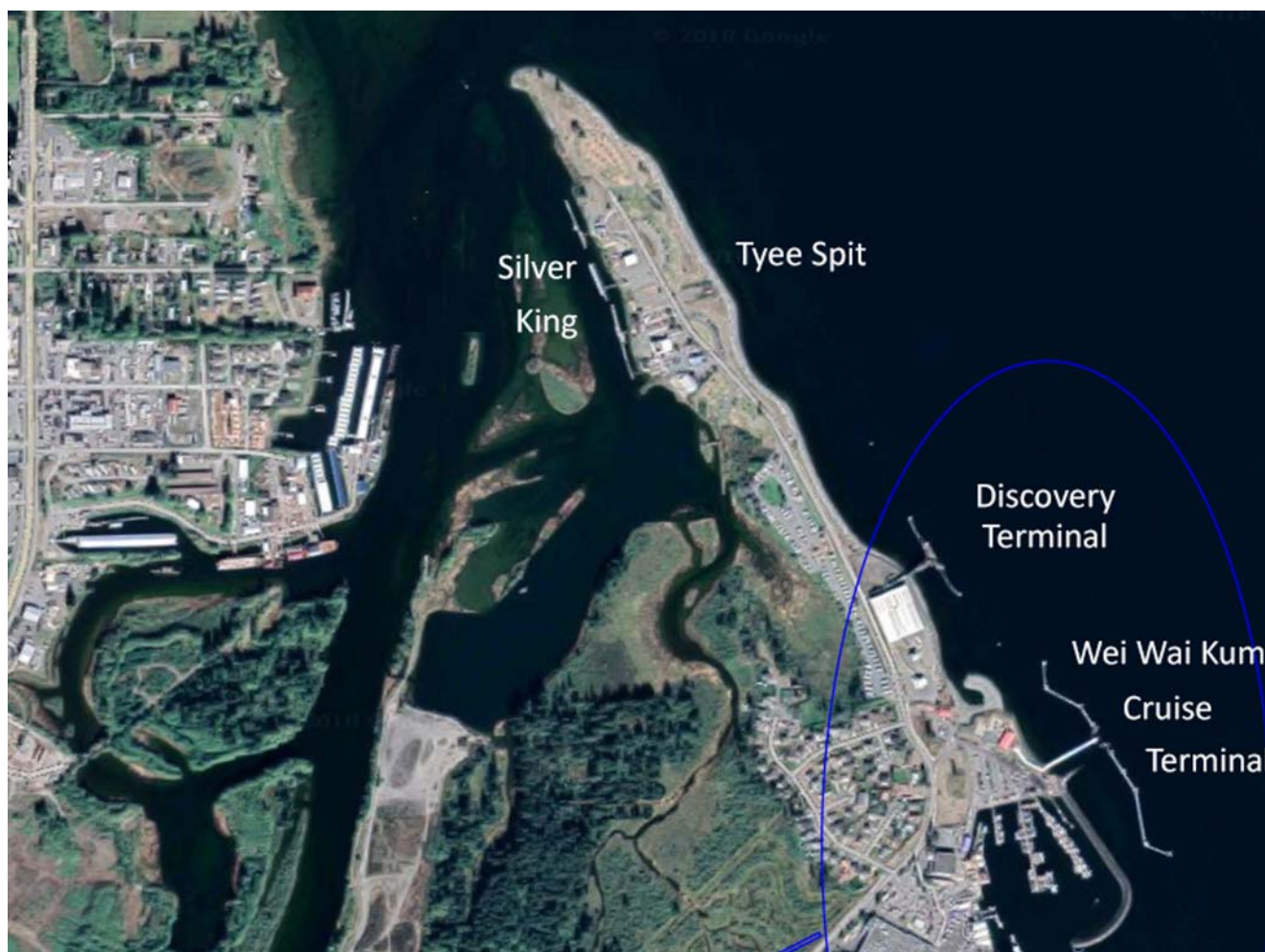
Port of Campbell River
