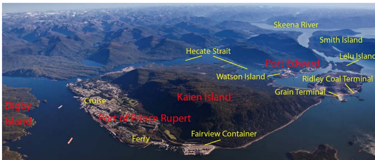
Prince Rupert Port—Port Edward—Ridley Island Grain and Coal Terminal
