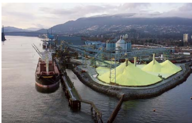
Vancouver Wharves Bulk Terminal
