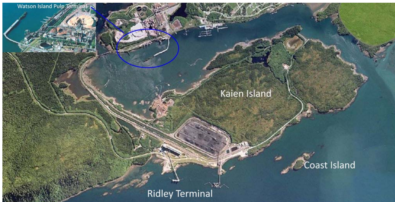
Porpoise Harbor—Watson Island Pulp Terminal
