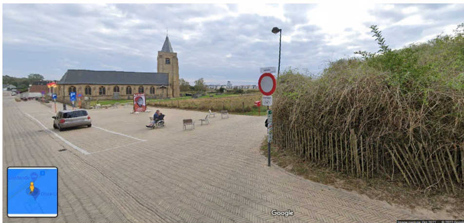
Figure 14: Position of the Parish Church of Our Lady of the Ascension (ID 4971) in relation to the modern frontage.
