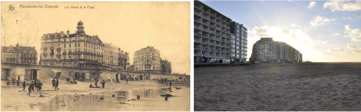
Figure 43 (left) Mariakerke Beach with hotels taken around 1900 (ID: 1024) ( https://nl.geneanet.org/prentbriefkaarten/view/7699848#0 Geneanet, Creative Commons (BY-NC-SA 2.0)), shows the beach level to be very low. Modern image on the right from Nov 2021 shows the beach levels much higher, the buildings have been replaced post-war and sand levels are being replenished to prevent erosion.
