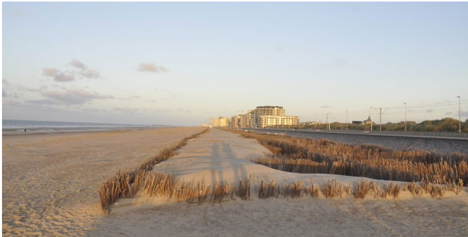
Figure 16 A section of dunes south of Zeedijk (Site: 5100). Taken November 2021.
