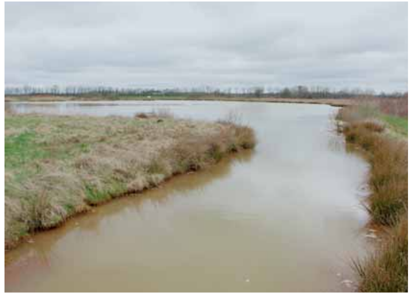
In ochre ponds the dissolved iron is oxidized on plants, and the ochre precipitates out.
