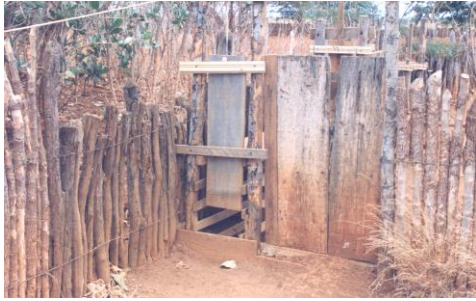
Figure 91: Guillotine gate entrance
