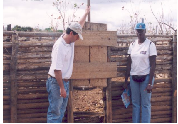
Figure 85: Use of Bamboo in Corral Construction and manual guillotine gate.
