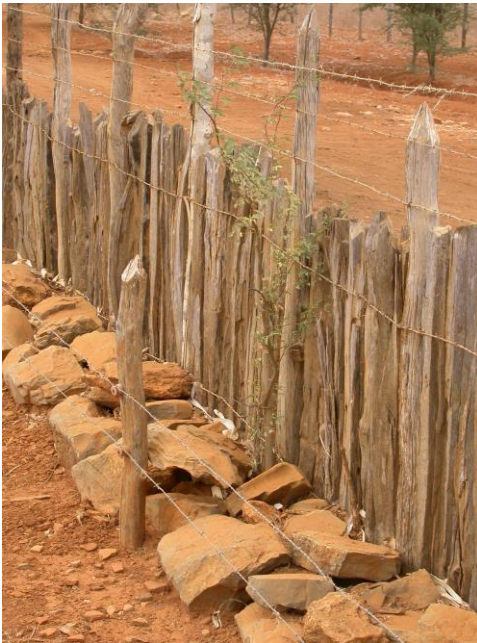
Figure 66: Wooden fence with electric fencing on the inside.
