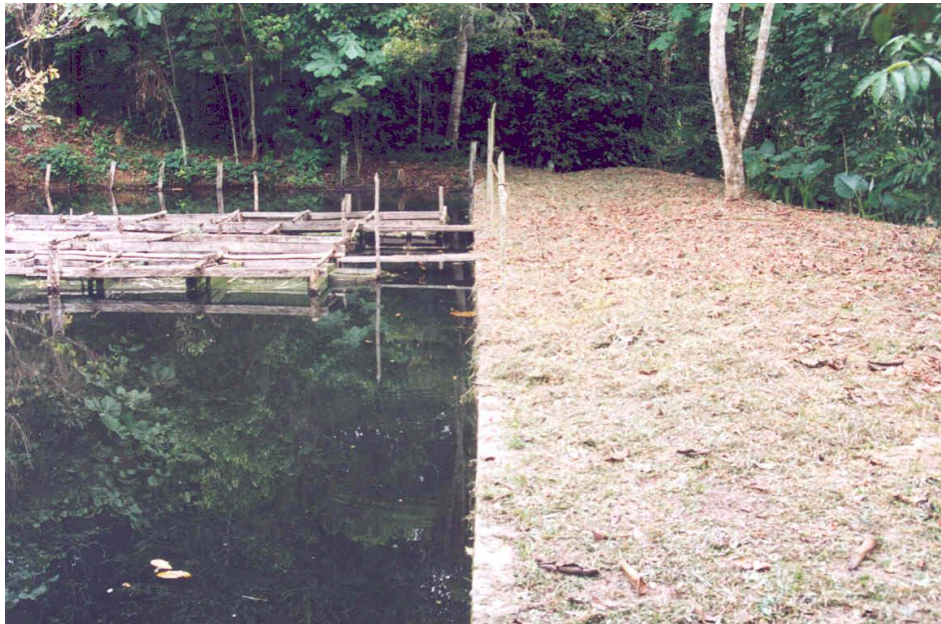
Figure 126: Side view of the pond or dam head made from an earth embankment and a row of concrete blocks.
