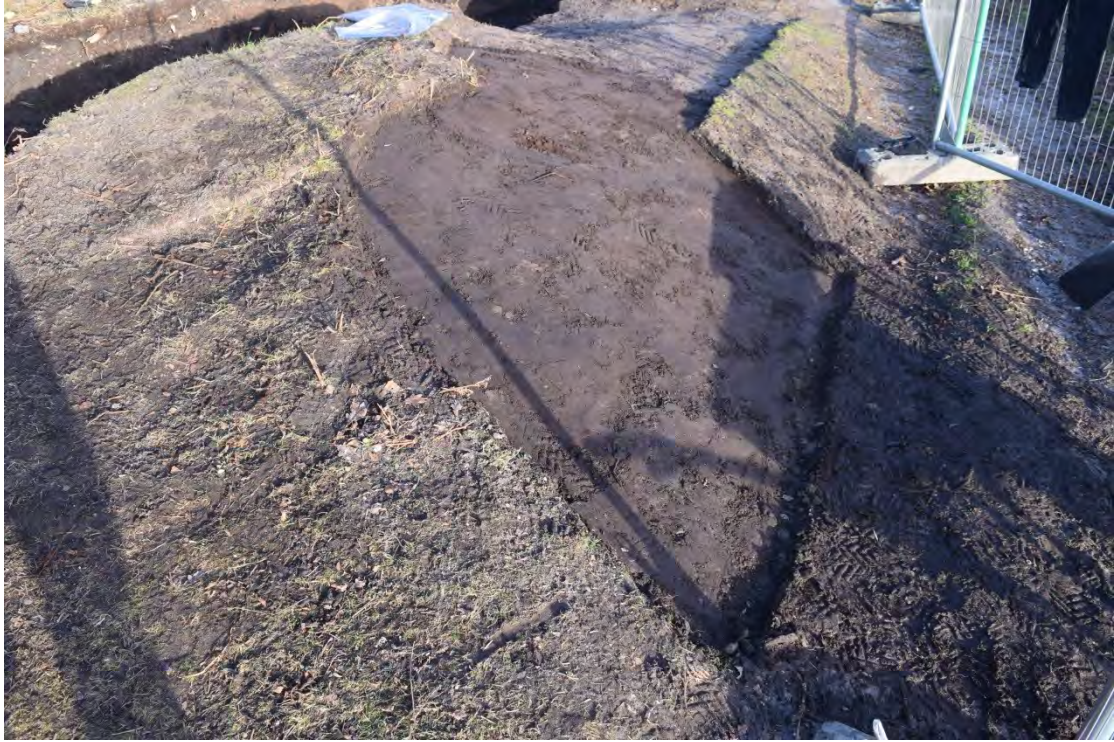
Plate 11 – Working shot showing re-profiling of western damaged area. Facing NE.
