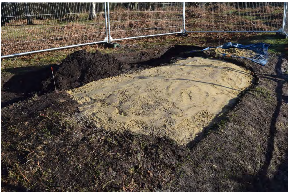
Plate 12 – Working shot showing re-profiling of eastern damaged area. Facing NE.
