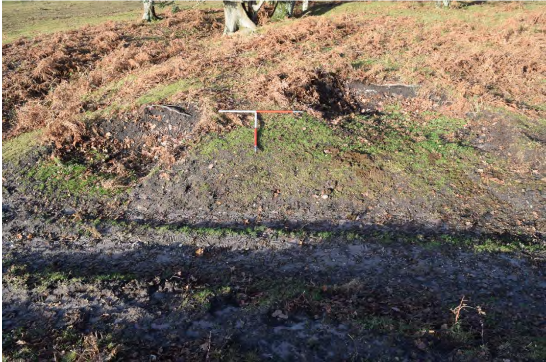
Plate 1 – View of damaged areas prior to reinstatement. Facing N, scale = 2x2m.
