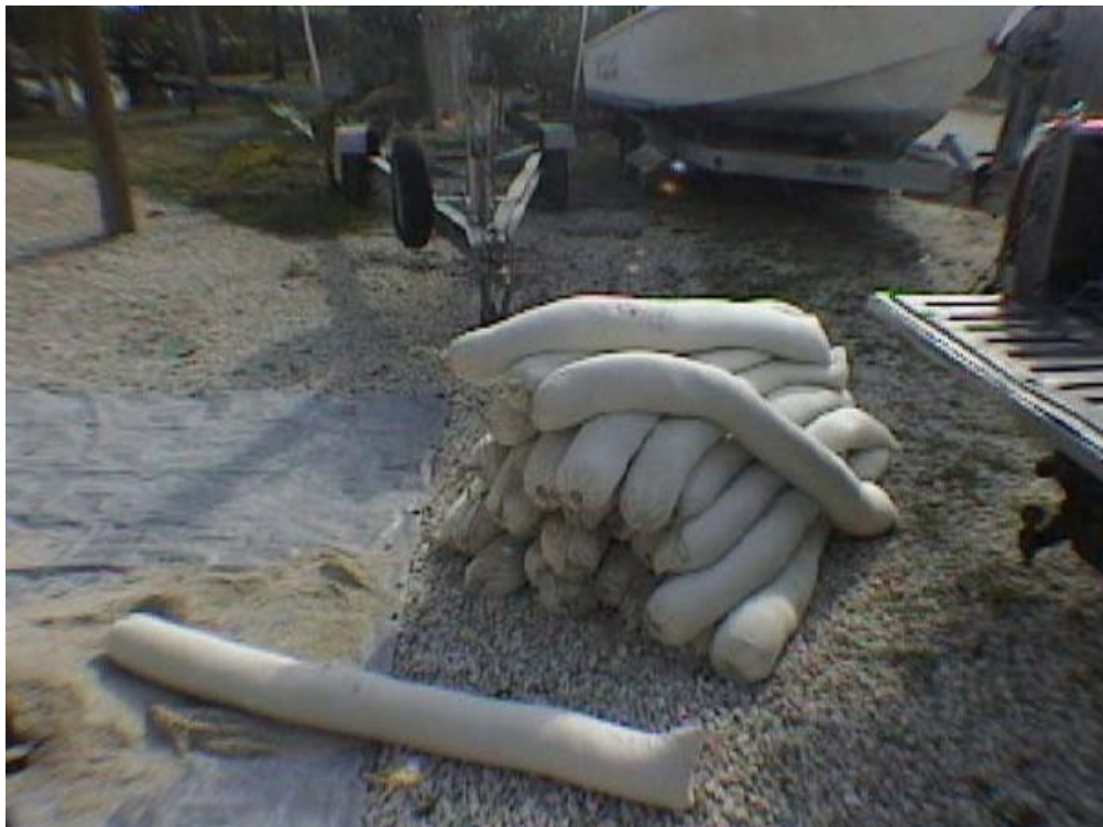
Figure 2. Filled sediment tubes ready to be deployed.
