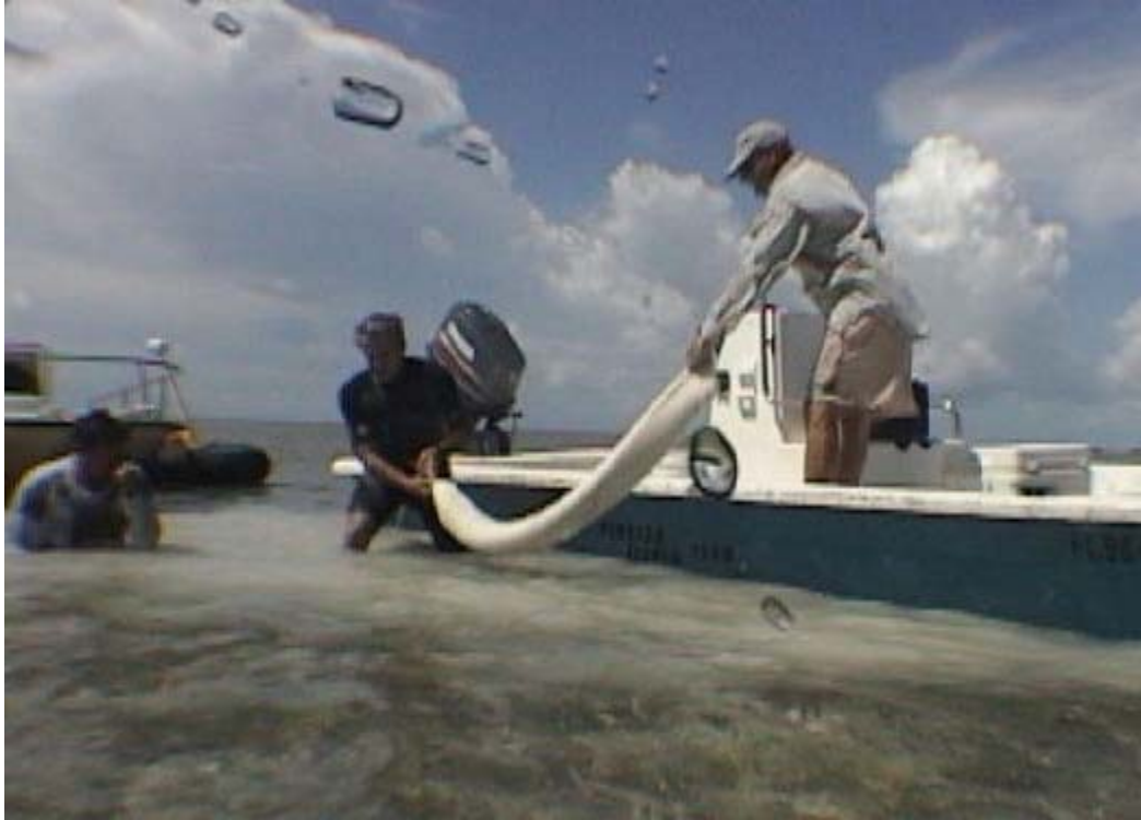
Figure 7. A shallow draft vessel was maneuvered close to the propeller scar and the sediment tubes were lowered into place.
