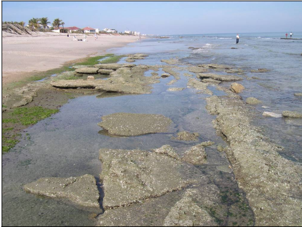
Figure 1.3. Broken pavement structure, nearshore hardbottom, central Brevard County, Florida. Photo by K. Lindeman.
