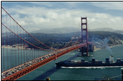
Large cargo ships daily transit the sanctuary enroute to and from the Port of San Francisco. Photo: NOAA
