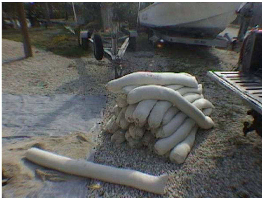
Figure 2. Filled sediment tubes ready to be deployed.
