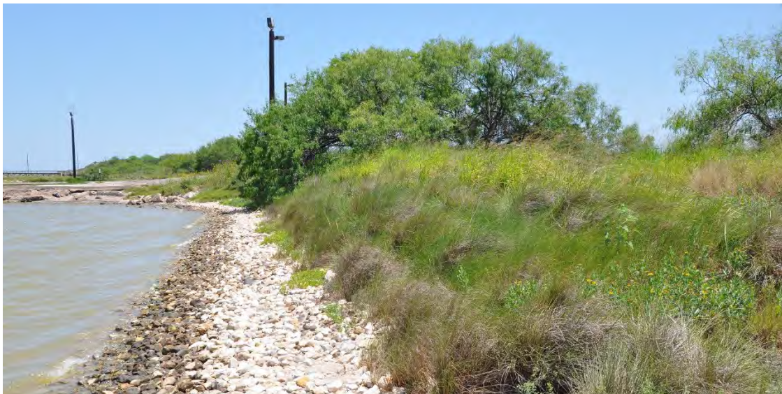
Gulf cordgrass, marshhay cordgrass, and seashore dropseed used on a shoreline erosion control project
