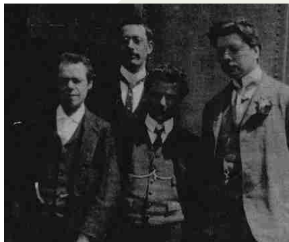
On the roof top of State Library 2nd and 3rd from left H. Wright and W. Ifould
