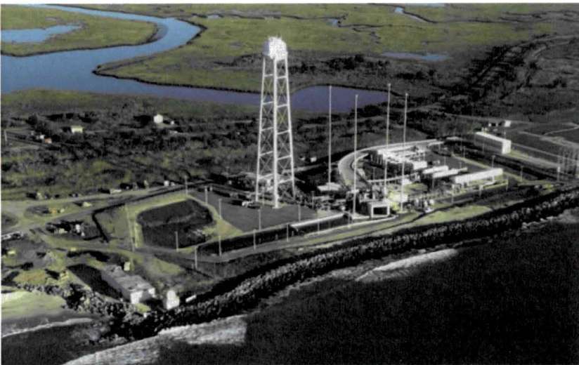
Launch Pad 0A at Wallops Flight Facility, VA. Pad systems are controlled by an integrated system designed and built by Command and Control Technologies Corporation and powered by Command and Control Toolkit.
