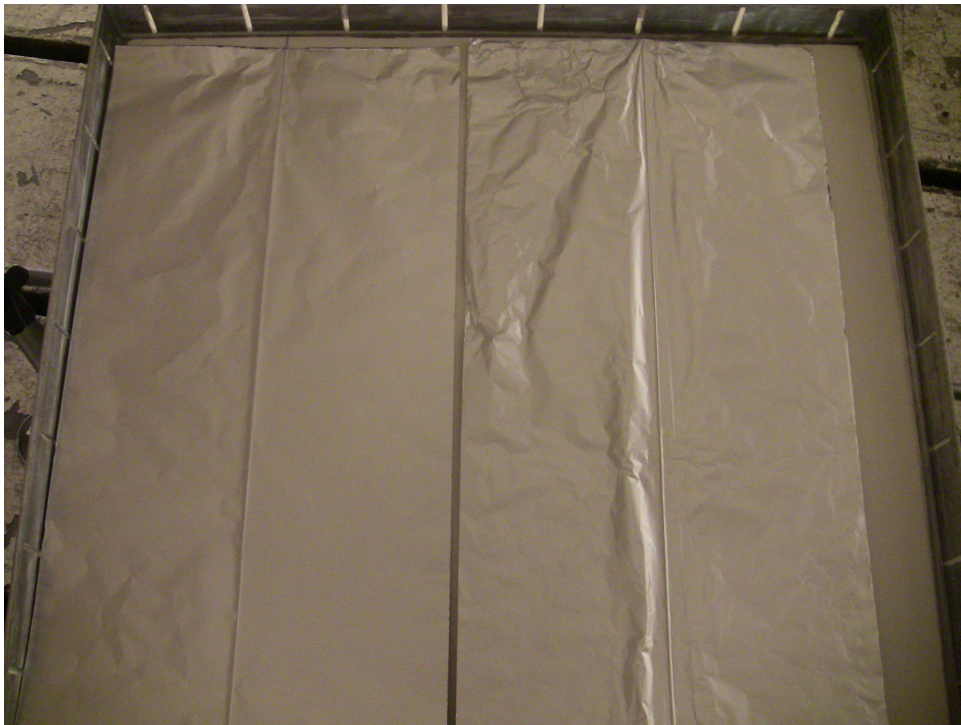
Figure 10. Standing Wave Marks Appeared on the Thin AL BAC Panel at Right, But Not on the Thick Panel at Left
