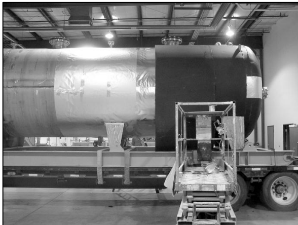
5. Inner vapor barrier plus first layer of foam.
