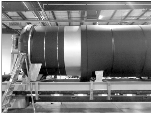
6. Final pass of middle vapor barrier with outer foam layer.
