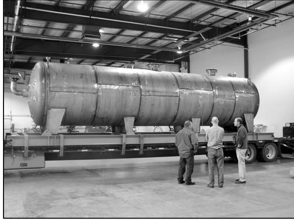
4. Liquid oxygen sub-cooler prior to insulation.
