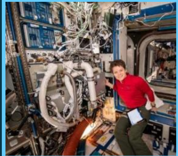
Thermal Amine CO 2 Scrubber
