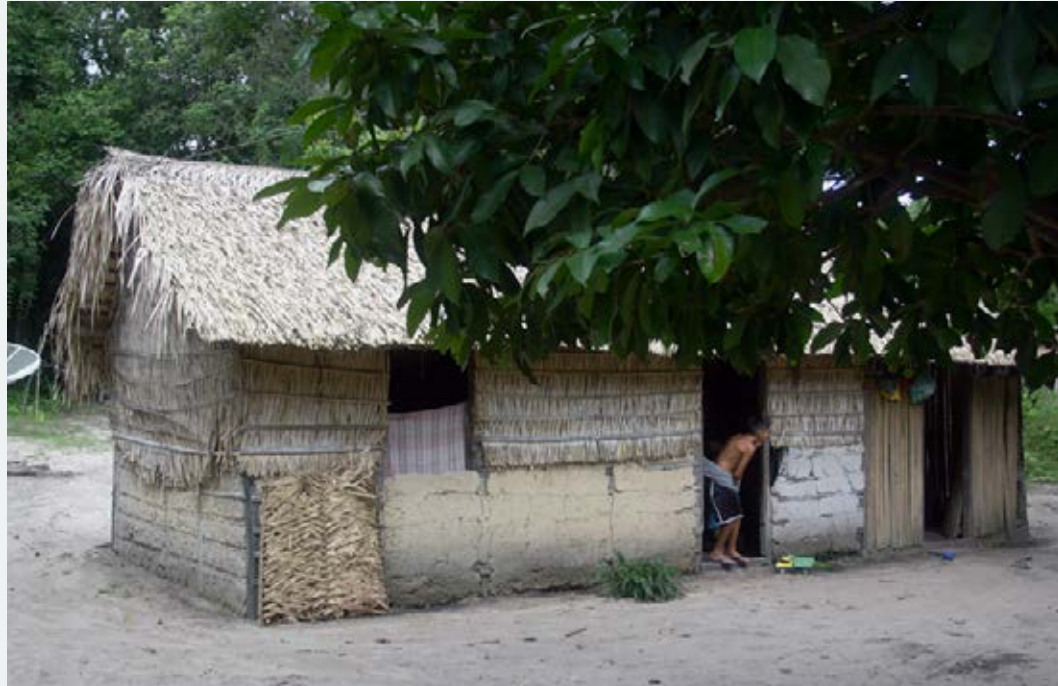
The use of mats as sunblinds is very suitable to the Amazonian region, since they are produced with natural materials that refrain light and heat.
