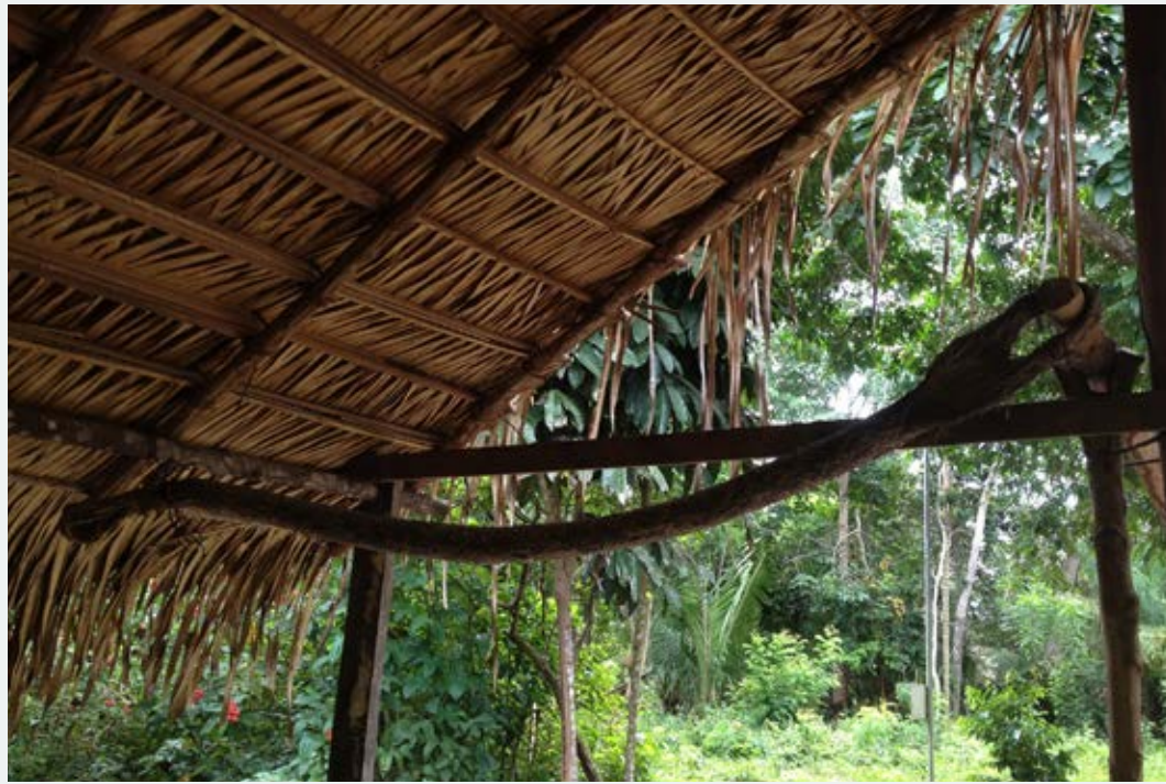
When not in use, the tipiti is kept hanging in the roof structure of the flour production house.
