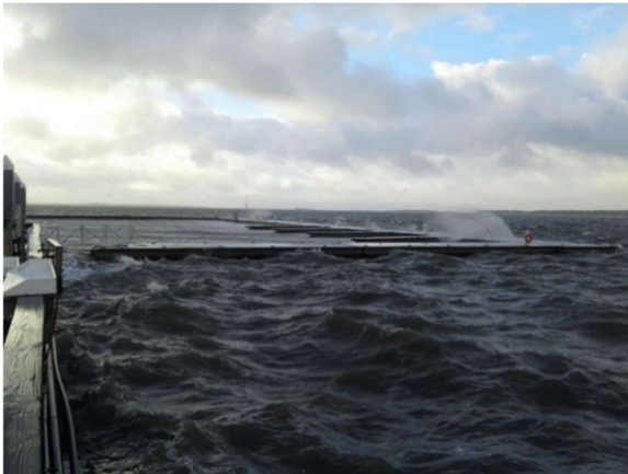
Floating Breakwater (Charleston, SC)
