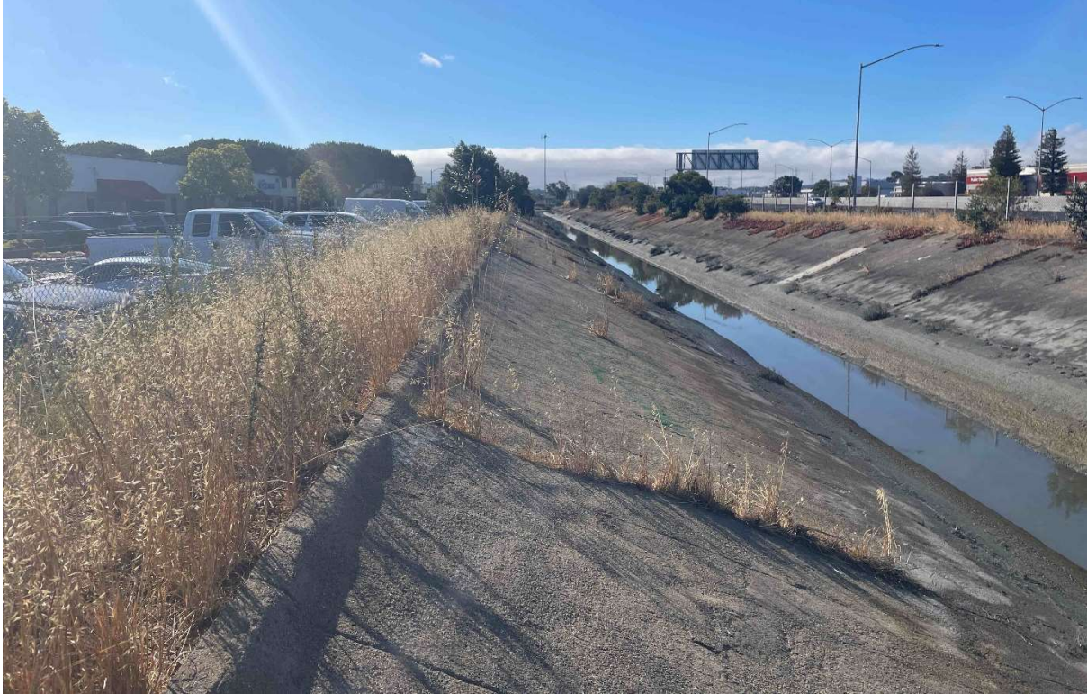
Photograph 27. View of concrete-lined Gilberth Canal. Photo facing southeast.
