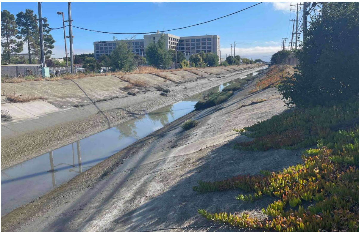
Photograph 26. View of concrete-lined El Portal Canal. Photo facing northeast.
