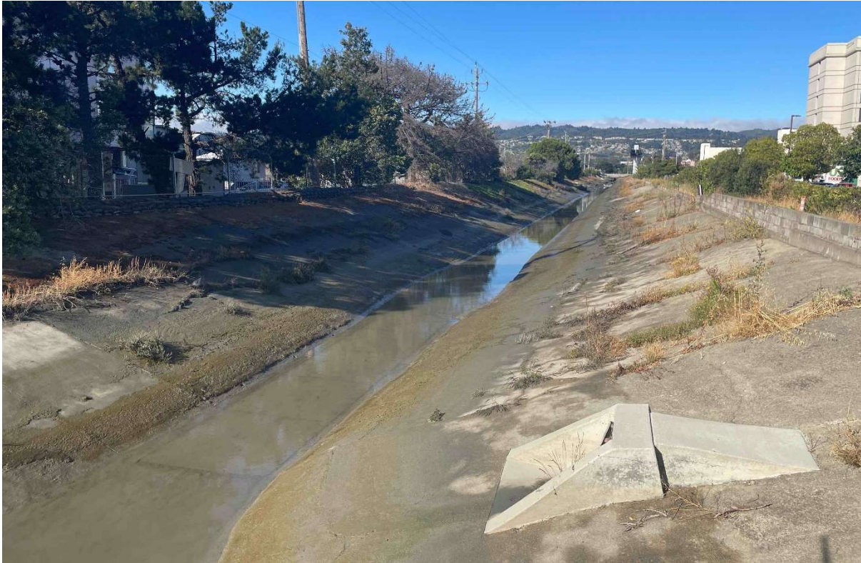
Photograph 25. View of concrete-lined El Portal Canal. Photo facing southwest.
