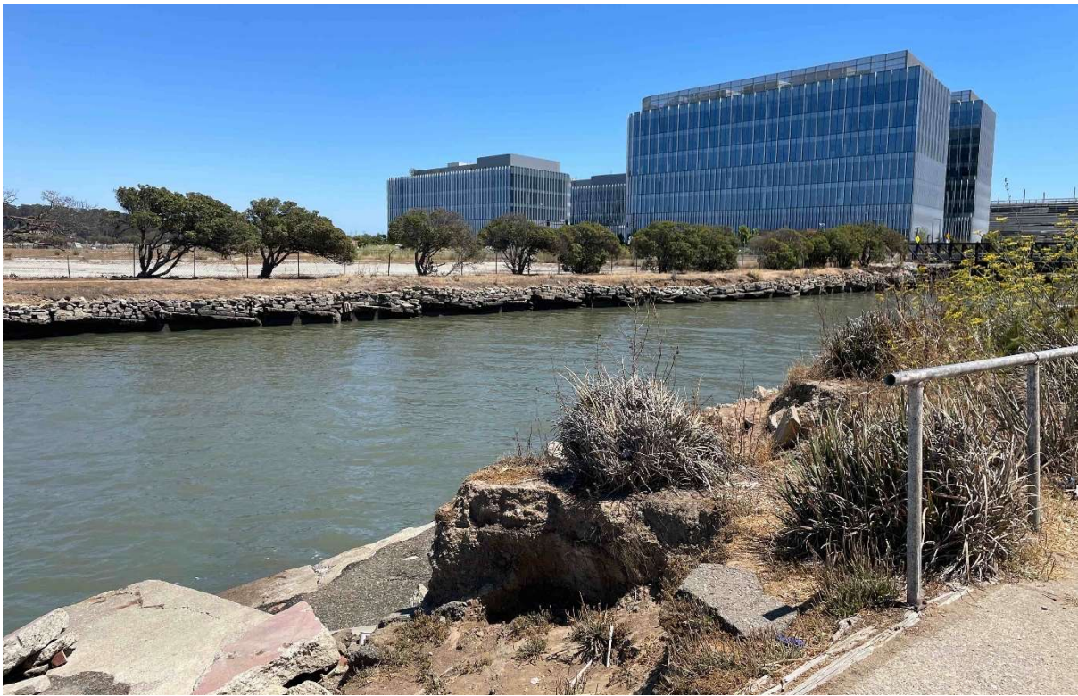
Photograph 42. View of the channel leading to Burlingame Lagoon. Photo facing southeast.
