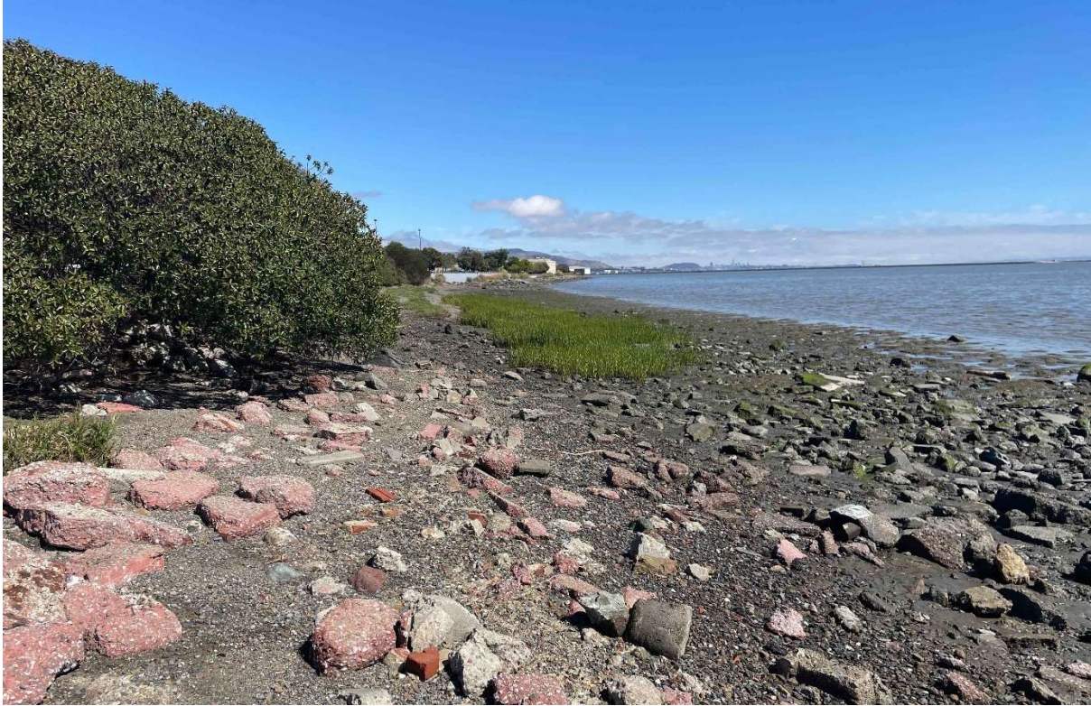
Photograph 31. View of rip-rap placed along the Burlingame shoreline. Photo facing north.
