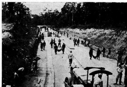
Figure 17. Construction Scene on Tamu-Kalewa Road in Burma
