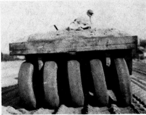
Figure 6. Static compaction with roller, rear-end view. (Five wobble wheels at rear end, four wobble wheels at front end.)
