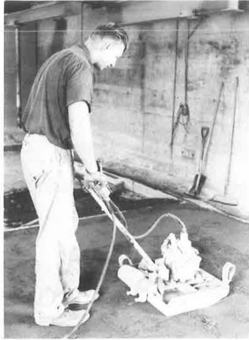
Figure 3. Final consolidation and leveling with vibrating sled.
