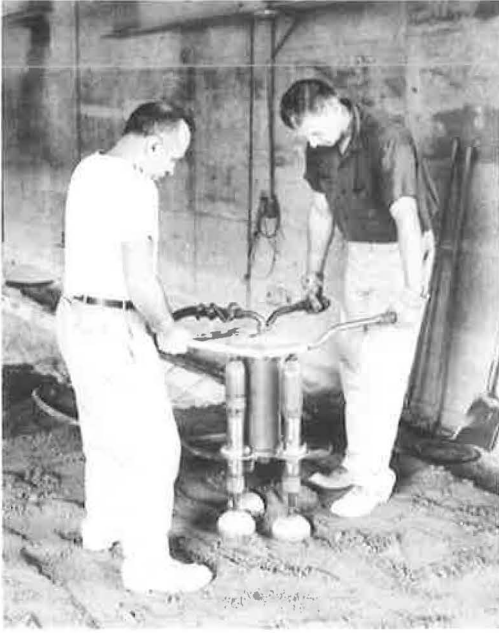
Figure 2. Consolidation of subbase with mechanical tamper.
