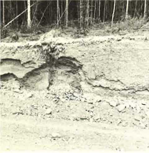
Figure 7. Erosion of vertical loess backslope due to runoff concentration.
