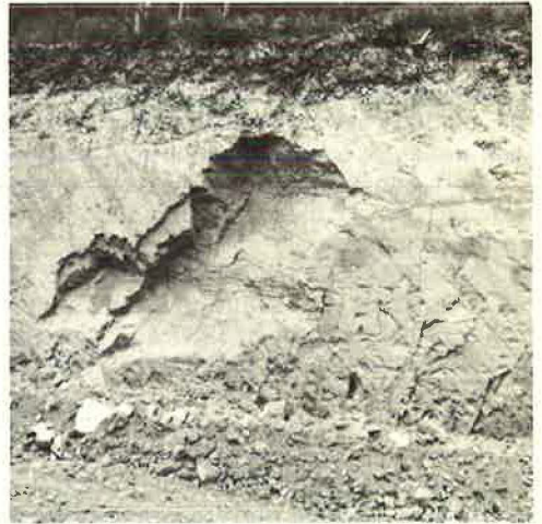
Figure 6. Chunking of vertical loess backslope.
