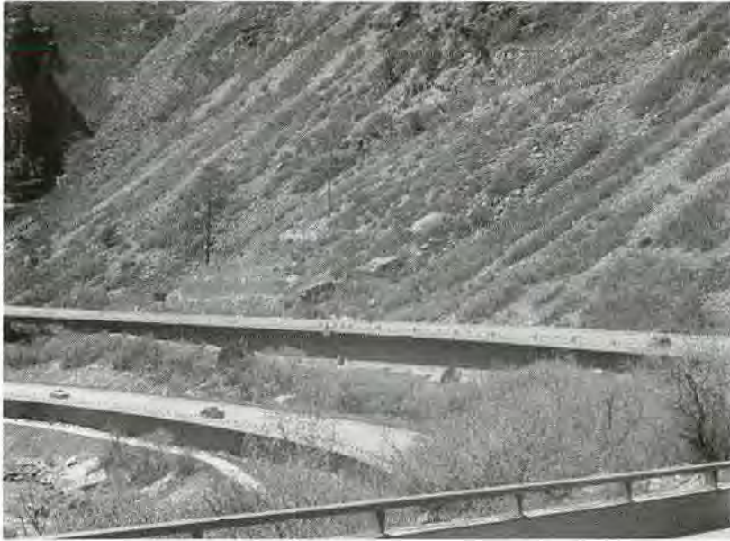
FIGURE 20-22 Completed Interstate-70 crossing extensive talus, Glenwood Canyon, Colorado.
