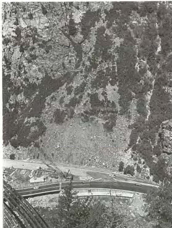
FIGURE 20-6 Multiple overlapping talus cones forming complex talus deposit, Glenwood Canyon, Colorado. Construction of Interstate-70 is under way at base of this deposit.
