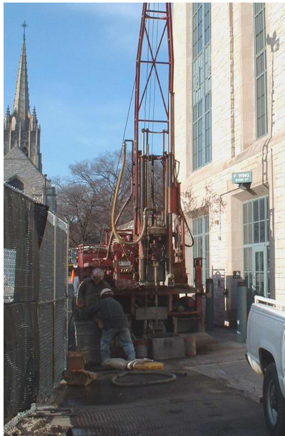
Inclinometer installed between a shored excavation and an existing building (Blackburn).
