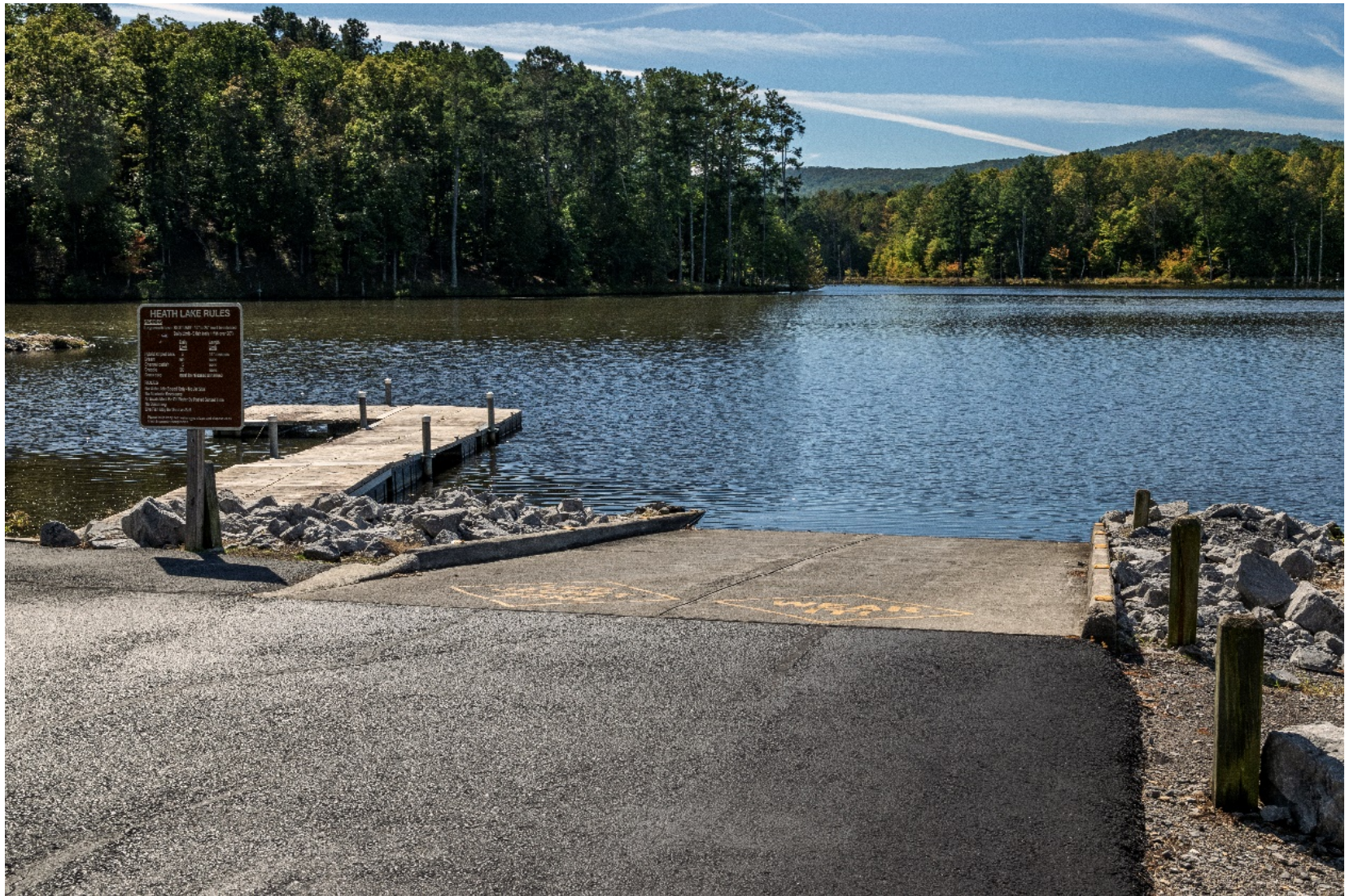
Figure 27 View of Auxiliary Pool II (Heath Lake) Boat Ramp
