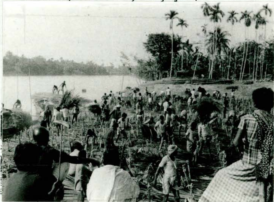
Filling mattress with reed and goalpata
