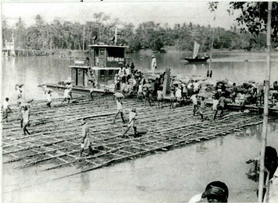
Ballasting of mattress
