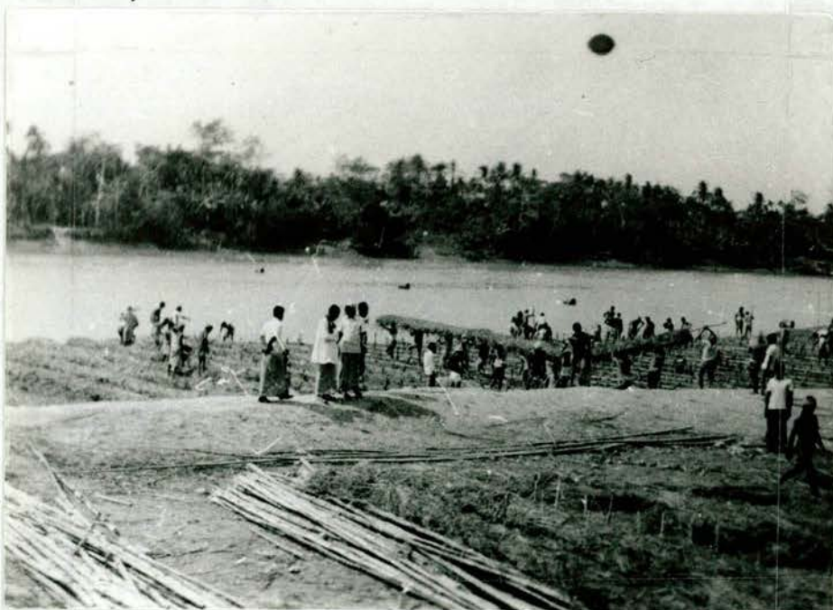
Sill mattress almost ready
