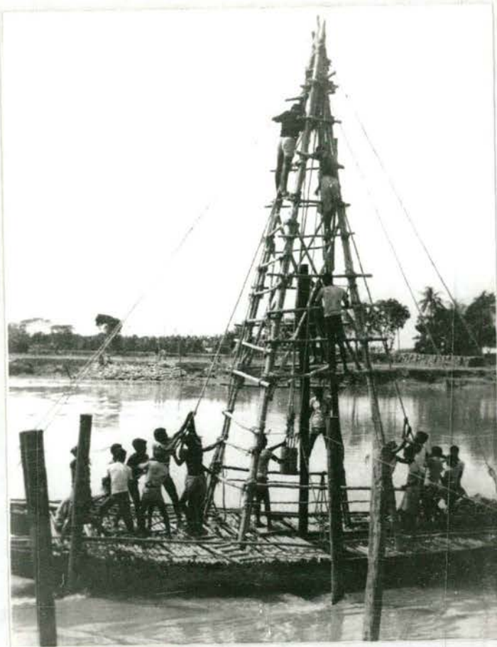
Pile driving for cofferdam bridge
