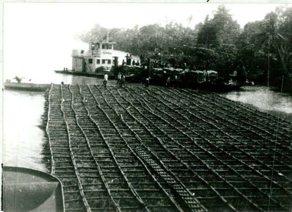
Positioning of mattress on sink location
