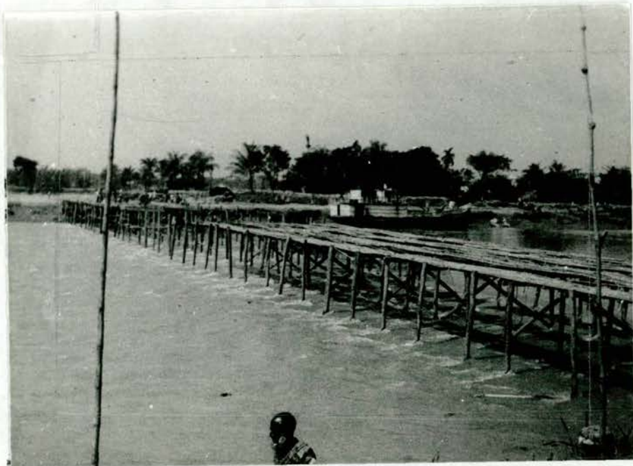
Finishing walkpaths and bamboo screen piling
