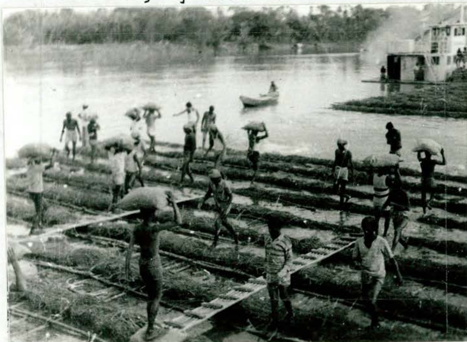
Ballasting of sill mattress
