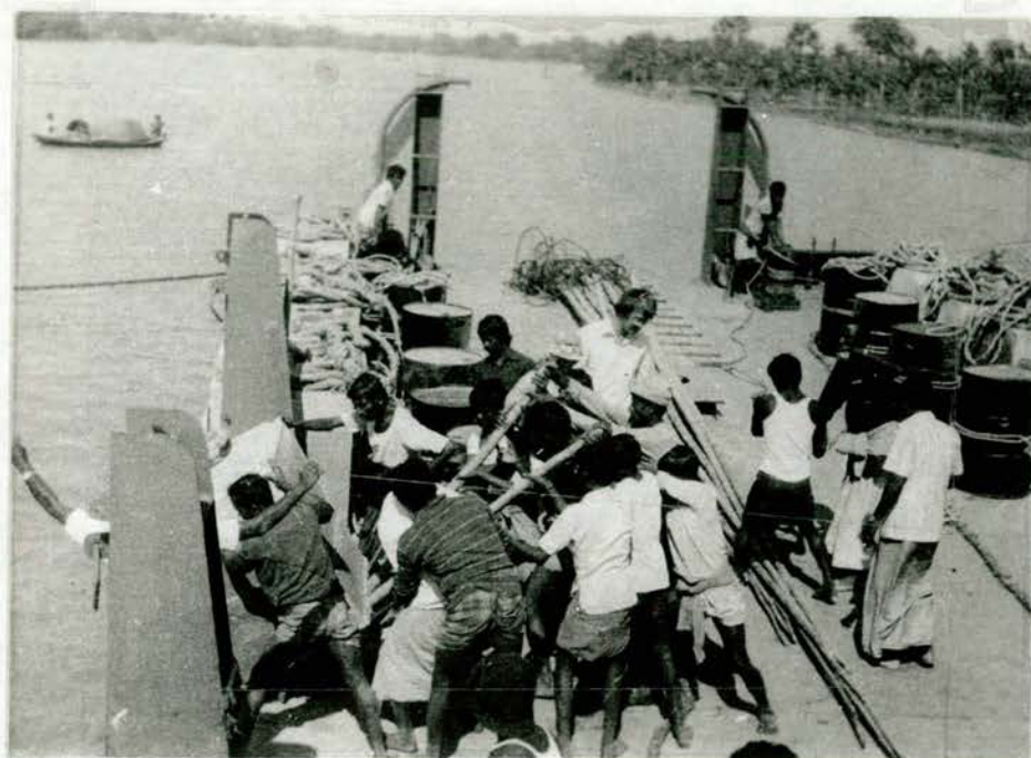
Placing anchor blocks in position
