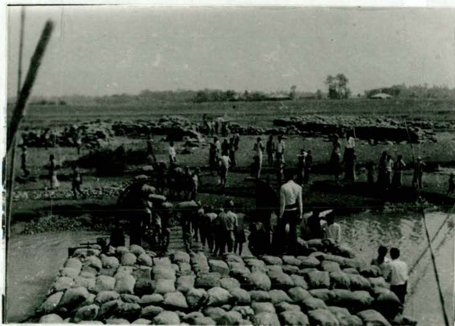
Filling and loading of gunny bags
