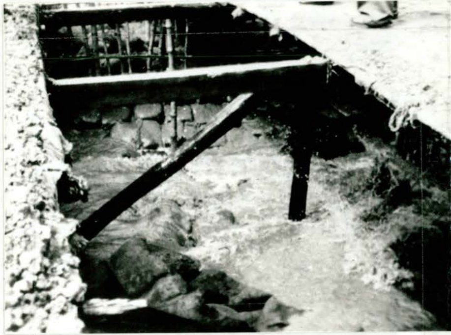
The final closure gap
