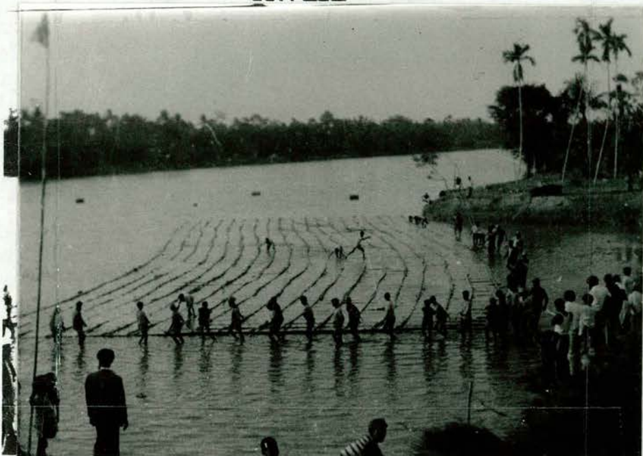
Turning the under grate in correct position
