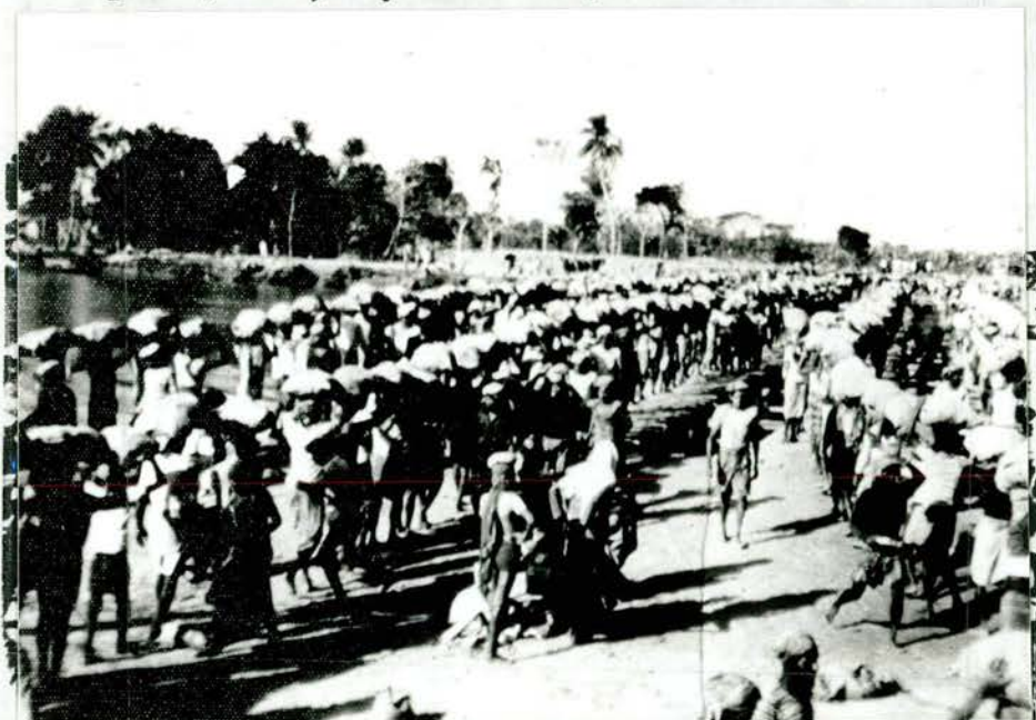
Dumping gunny bags over four walkpaths by 1600 labourers
