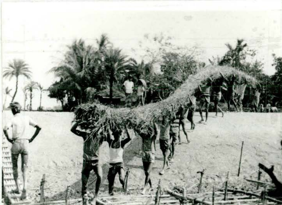
Carrying reed roll to sill mattress
