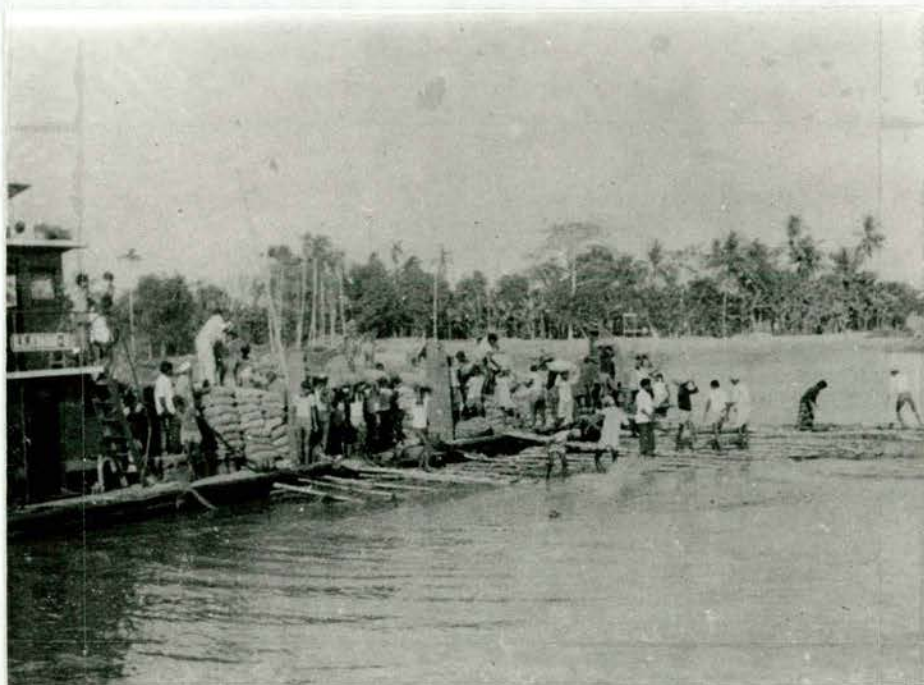
Ballasting by head load almost ready
