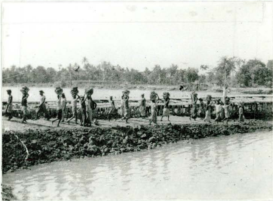
Earthwork in progress
