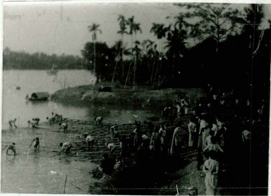
Carrying under grating to submerged terrace
