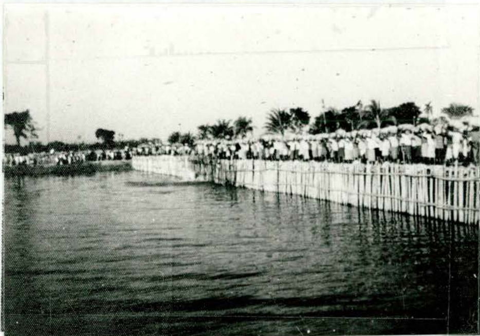
Start final closure operation, dumping gunny bags from walkpaths
