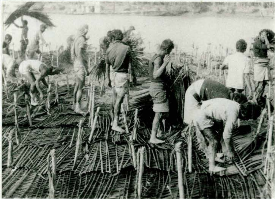
Marking middle layer of goalpata leaves
