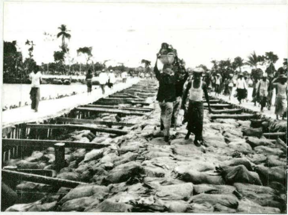
Gunny bag dam upto PWD + 8 ft. middle walkpaths already removed
