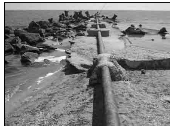
(4) Wastewater pipe laid upon a groin (Tomis)
