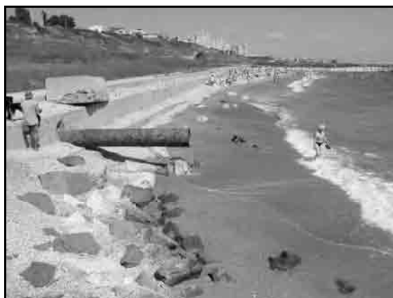
(3) Wastewater pipe opened to the beach (Tomis)
