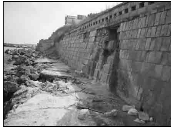
(2) Outfall of wastepipe at north Eforie Nord
