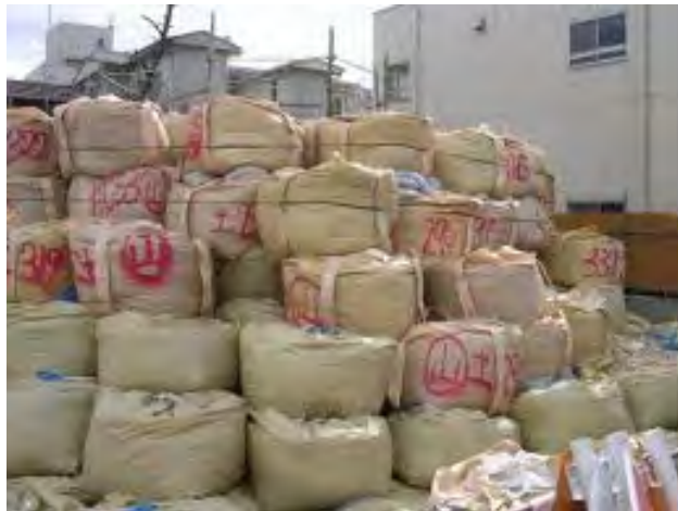
Figure 5.2.12 Sand Bags as Counterweights as a Landslide Countermeasure (source: JET)
