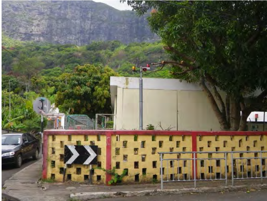
Figure 6.2.15 Installation of the Early Warning and Evacuation System in Chitrakoot (source: JET)
