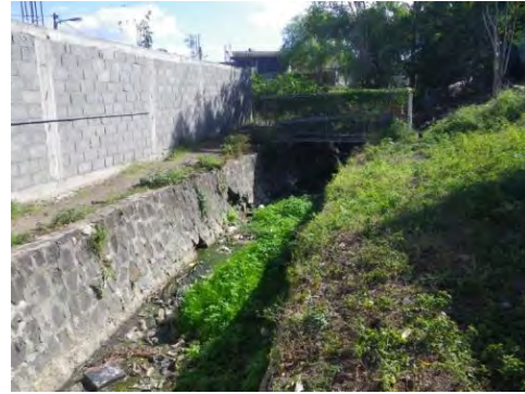
Photo 5.2.4 Seen above the Blockage No deformation can be seen.
