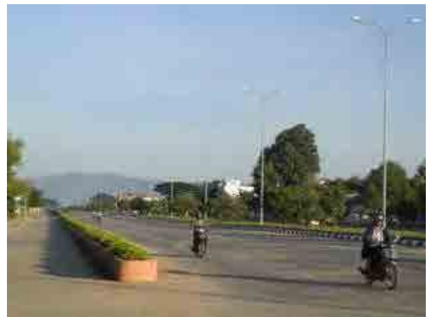
Street lights without overhead service wire
