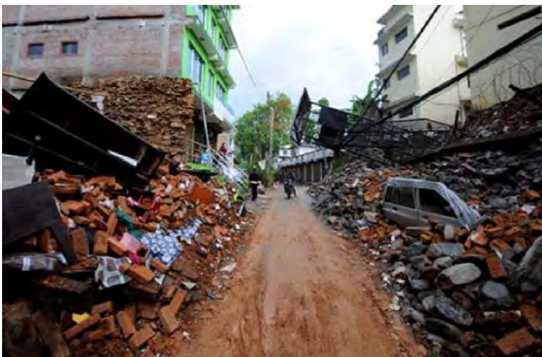
Picture 3.13 Collapsed Private Buildings in Sindhupalchowk District
