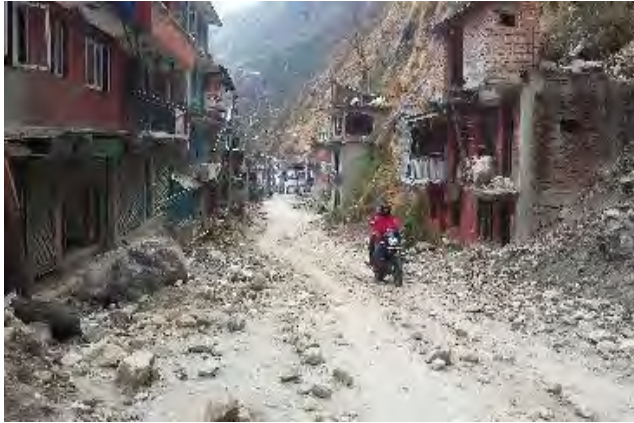
Picture 3.9 Road Condition after the Earthquake
