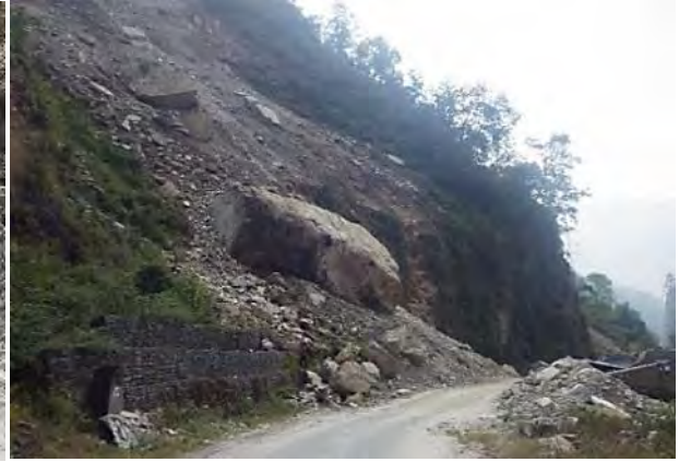
Picture 3.10 Landslide Hit Highway
