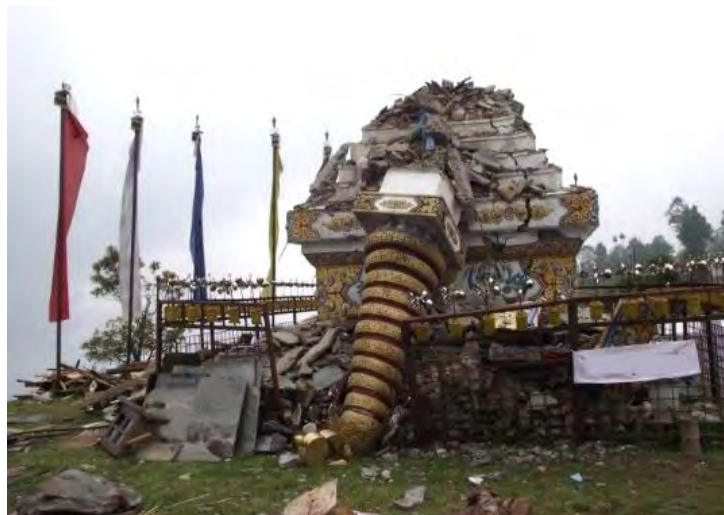
Picture 3.11 Collapsed Monastery
