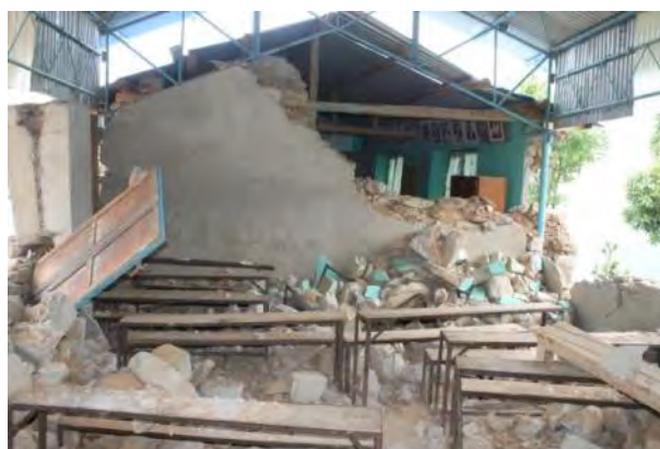
Picture 3.7 Collapsed Classroom in Sindhupalchowk District
