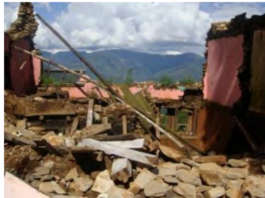
Picture 3.4 Collapsed House (Chautara)
