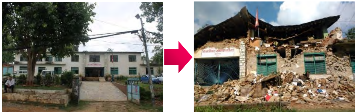
Picture 3.8 Earthquake Damage to DDC Office (Left: Before the Earthquake, Right: After the Earthquake)
