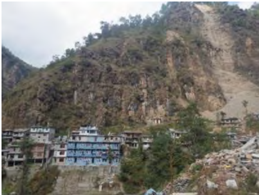
Picture 3.3 Landslide by the Earthquake (Marming)
