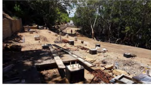
Hill Side Bungalows (HSB) type B number O1 and O2 completed for concrete foundation works
