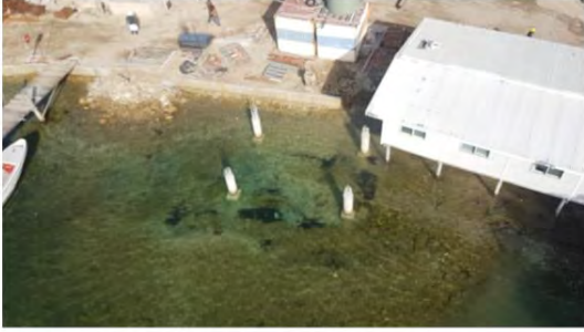
Dive Shop Foundation completed
