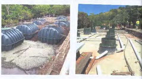
Installation of Sequencing Batch Reactor Plumbing System
