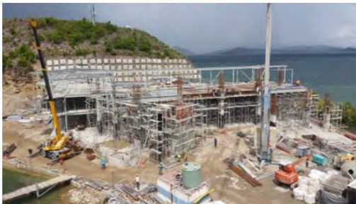
UPDATE ON CONSTRUCTION
