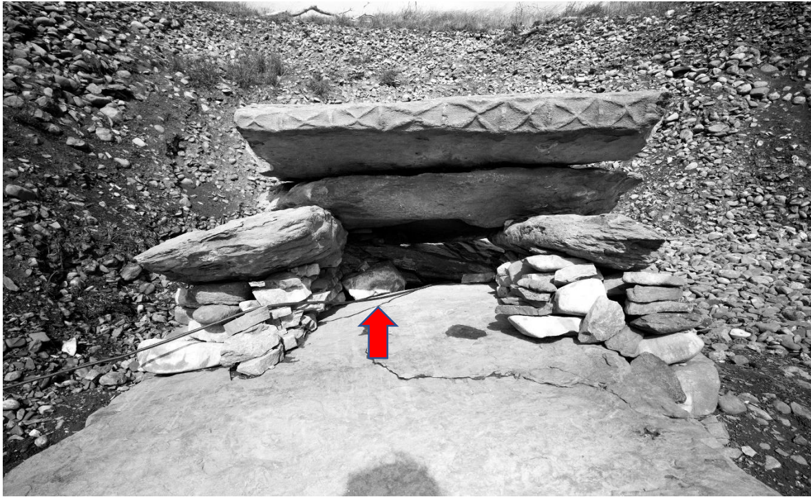
Figure 5-6 The roof-box at Newgrange prior to restoration. The quartz block (indicated by the arrow) was still in place at this time © Photographic Archive, National Monuments Service, Government of Ireland
