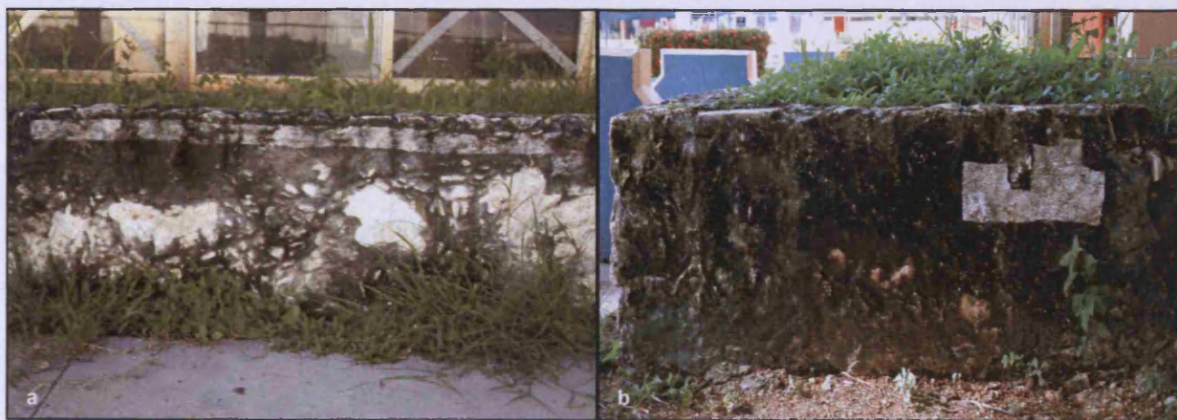
Figure 15 Sampling sites with partially removed biofilm Partially removed biofilm on a: the sun-site at the south-facing part of the wall and b: the shade-site at the east-facing part of the wall.
