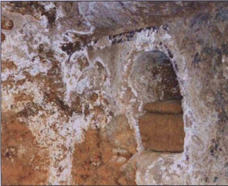
Figure 8 Salting on tomb of Servilia Salting on the internal walls of the tomb of Servilia, Carmona, Spain. Picture by C. Gaylarde.
