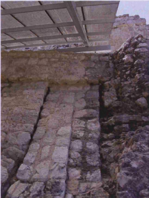
Figure 49 Protective roof on a north wall at the Mayan pyramid of Edzna, Mexico. Directly underneath the roof (left), where rain protection was the best, very little microbial biofilm developed. Underneath the final, less protected metre of the roof (middle) more biofilm formation could be noticed and in completely unprotected areas (right) severe development of biofilm was visible.
