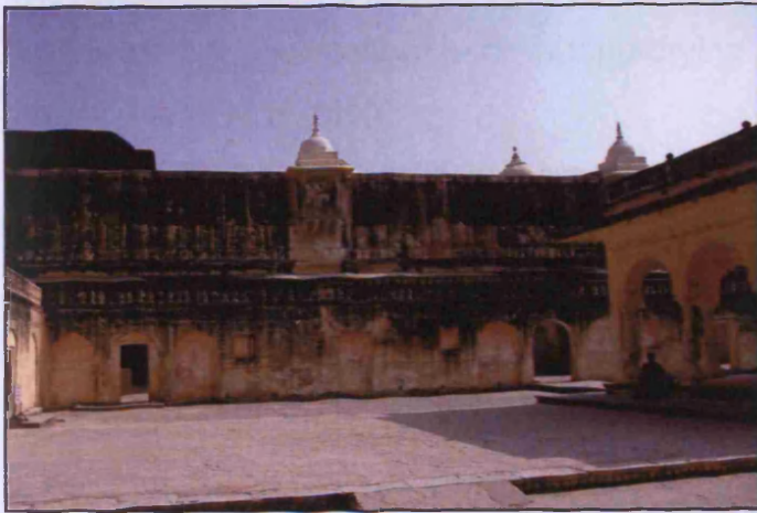
Figure 4 Ambar Fort Black biofilms on the surface of the Ambar Fort in Jaipur, India. Picture by C. Gaylarde.
