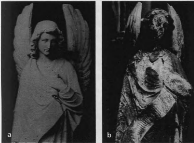
Figure 1 Biodeterioration of an angel statue The influence of biodeterioration on an angel statue of the cathedral of Cologne (Germany) photographed 1880 by Anselm Schmitz, Cologne (a) and 1993 by Dombaumeister Prof. Dr. A. Wolff, Cologne (b) (Warscheid & Braams, 2000).
