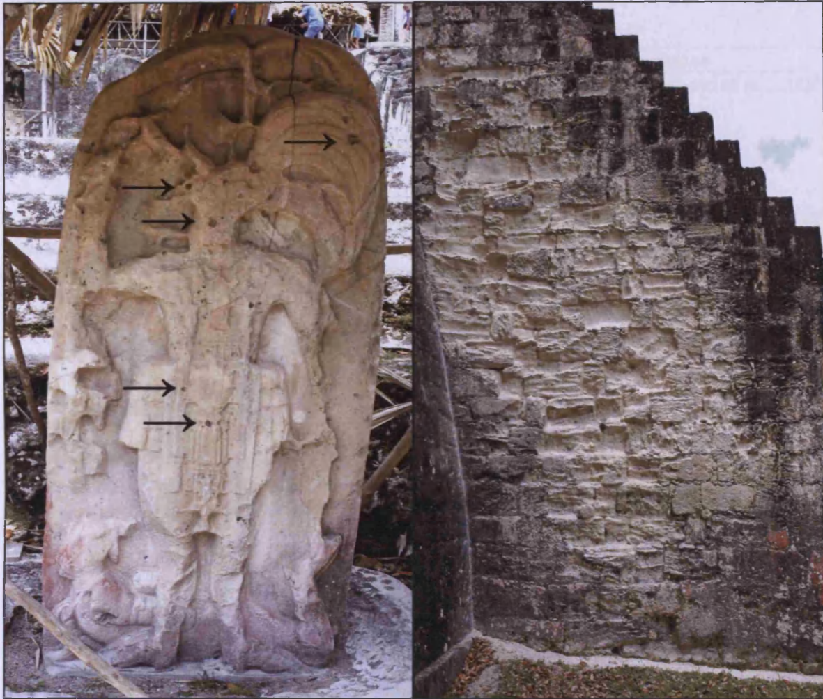
Figure 13 (left) Limestone statue showing erosion and pitting Limestone statue in Tikal, Guatemala showing severe cases of erosion and pitting (arrows). Figure 14 (right) Limestone wall showing exfoliation Limestone wall in Tikal, Guatemala with large areas of material loss in the surface due to exfoliation.
