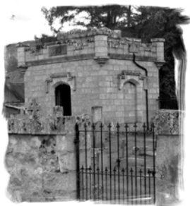
Vault in Braemar Cemetery
