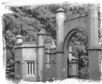
Cortachy Castle Gate House
