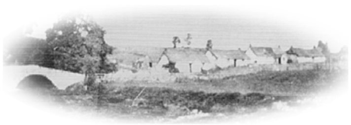
Pipe Hole, Glengairn
