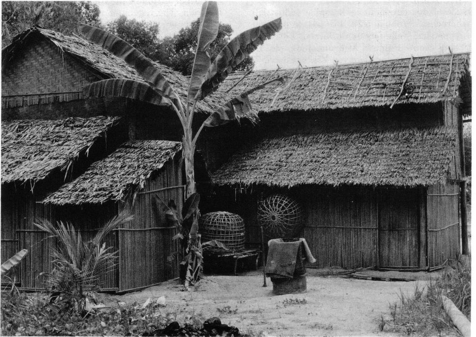
1. A village house near Trang, S. Thailand. The roof is thatched with Nypa leaflets; Walling is constructed from Salacca wallichiana petioles as are the hen coops.
