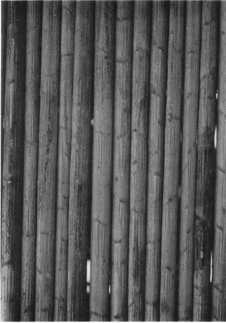
2. Salacca petioles, spines removed, nailed on a framework, make an airy wall; note the scars where spines have been removed.
