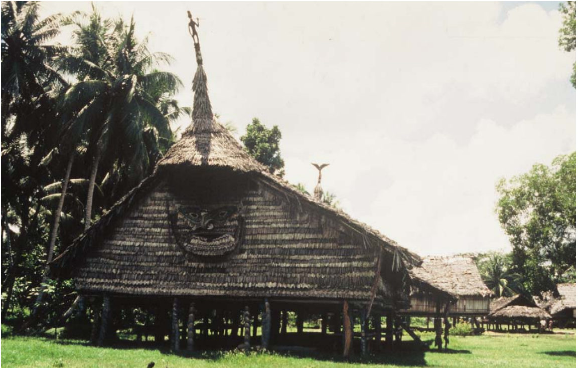
3. The "Spirit House" in Maramba Village. More than 20 canoe loads of Borassus leaves were brought the long way down the Sepik River to built the house in the traditional ways of the ancestors. Large parts of the roof and the pale parts of the walls was constructed with Borassus leaves, and for the rest, sago leaves were used.
