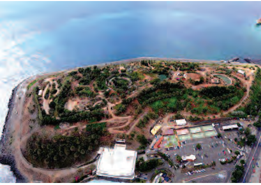
1. This aerial view of late 2010 shows the major construction works finished in 2011. Source: Palmetum archives.
