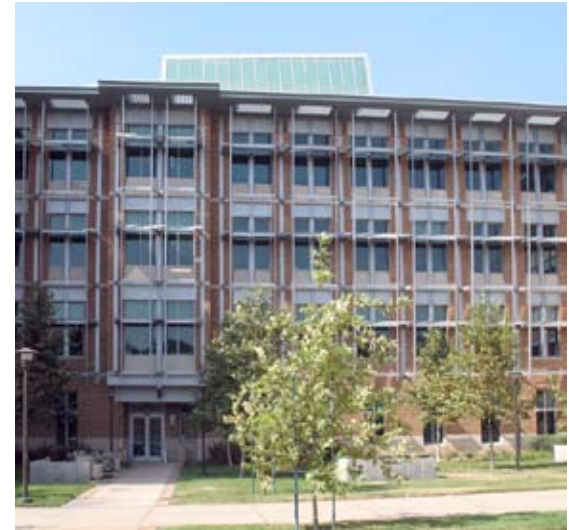
Physical Sciences Building: Louvered Sun Shades
