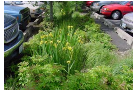
Stormwater Detention Swale
