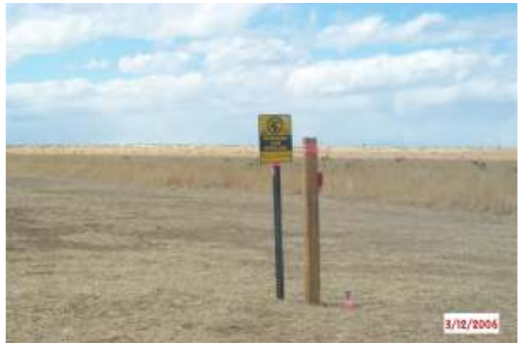
Gas Pipeline north of Mesa de Maya, on the western Carrizo Unit of the Comanche.
