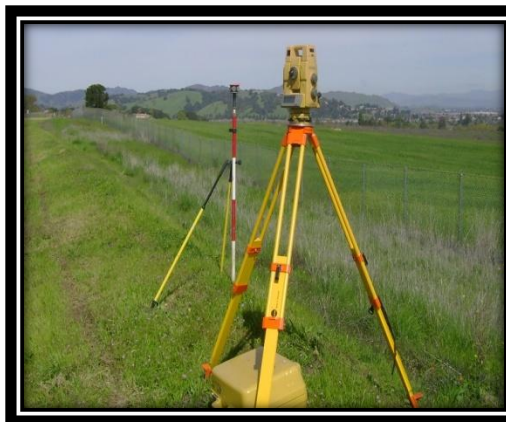
Surveying equipment-theodolite on tripod
